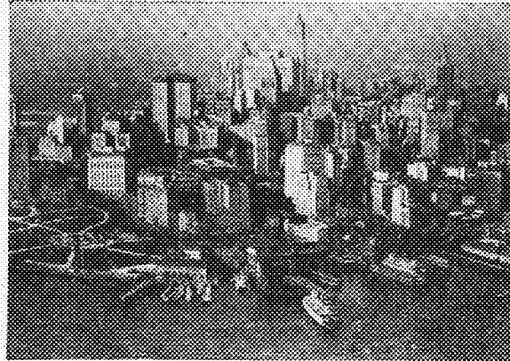
© Hamilton Macaulay, Inc., N. Y. OVER FIFTY OF THESE LARGE BUILDINGS REST ON FOUNDATIONS BUILT BY THE FOUNDATION COMPANY IN NEW YORK
