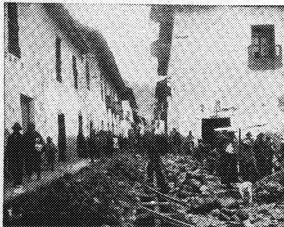
WATER PIPES BEING LAID BY THE FOUNDATION COMPANY FOR THE MUNICIPALITY OF CUZCO, PERU
