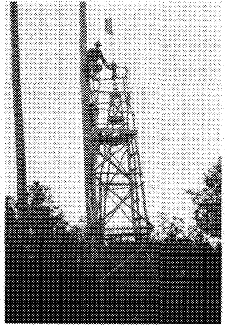
TRIANGULATION STATION "TOWER" The instrument is 18 feet above ground and allows sights to be taken for miles around. Ed Witt is seen testing the stresses in the framework.
