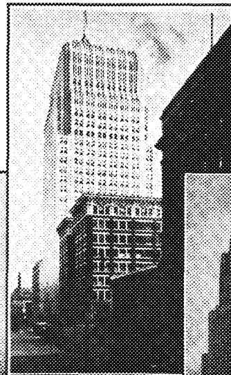
Pacific Telephone & Telegraph Company, San Francisco, Cal. J. R. Miller, T. L. Pflueger & A. A. Cantin, Associate Architects
