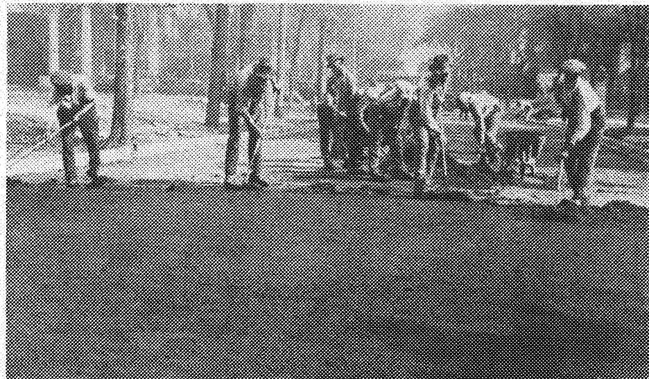
SPREADING THE ASPHALT SURFACE
