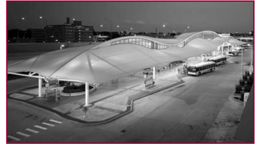
This Michigan transit station features a “green” roof that reduces runoff and maintains the building’s temperature.
