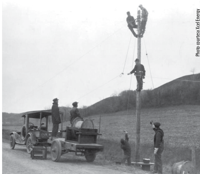
Workers put up the first power poles near Red Wing, Minn., in 1923.
