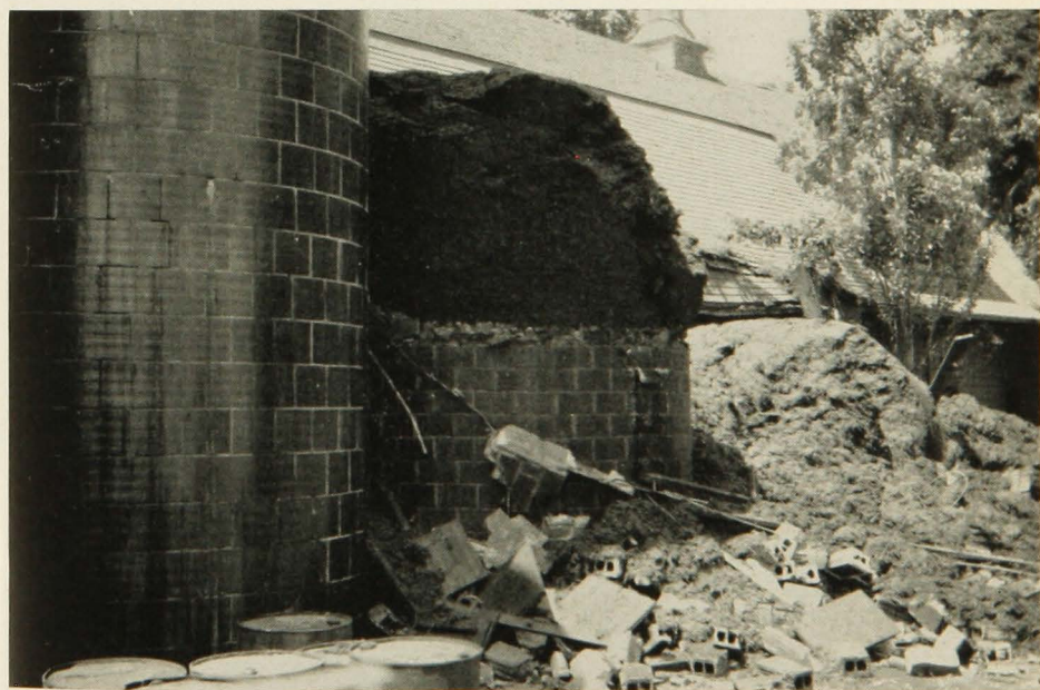
FIG. 8. THE REINFORCING OF OLD SILOS SHOULD BE CHECKED CAREFULLY. ADD OUTSIDE BANDS IF NECESSARY. THIS SILO COLLAPSED DUE TO THE PRESSURE OF ALFALFA SILAGE
