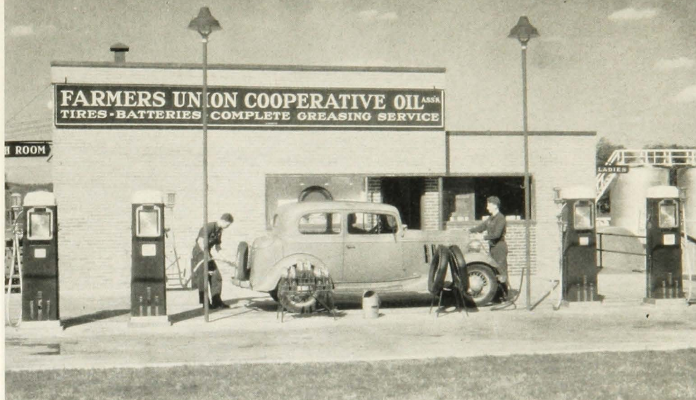
FIG. 7. SERVICING A CAR AT A COOPERATIVE STATION
