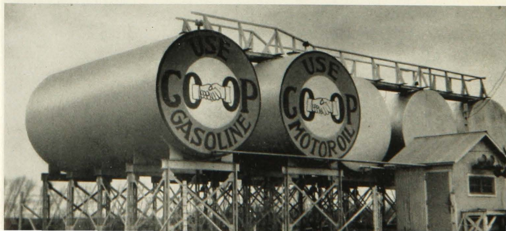
FIG. 12. TYPICAL BULK PLANT FACILITIES OF A MINNESOTA OIL ASSOCIATION
