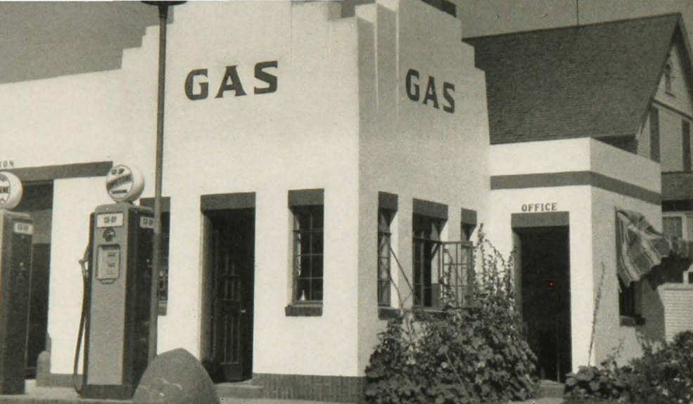
FIG. 11. AN ATTRACTIVE COOPERATIVE SERVICE STATION
