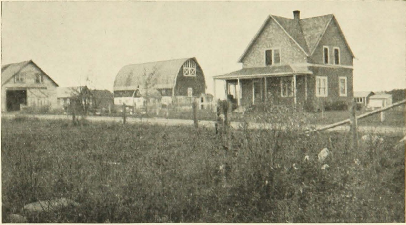
FIG. 22A. TYPICAL, FULLY DEVELOPED FARM IN THE RELOCATION AREA
