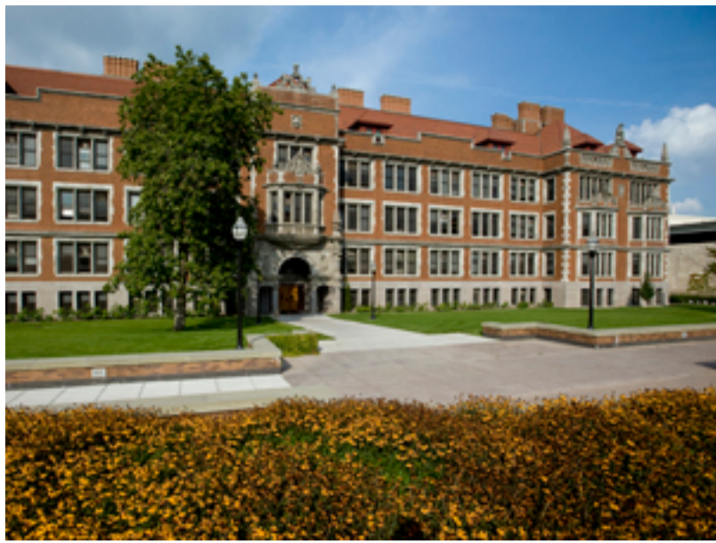
Folwell Hall in 2009, prior to the completion of a $34.5 million interior renovation.
