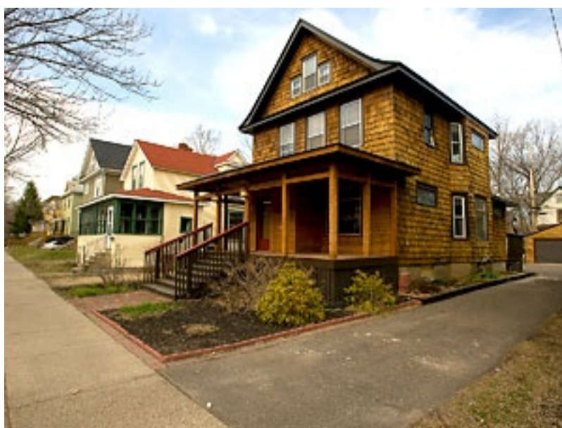
This house at 1022 16th Ave. SE is midway through its renovation (with gutted kitchen) and is open during the home tour. The University District Alliance bought the option on this home and it is for sale to an owner occupant.
