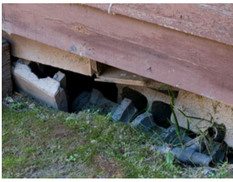
This crumbling cabin foundation is one reason the Itasca station needs attention.
