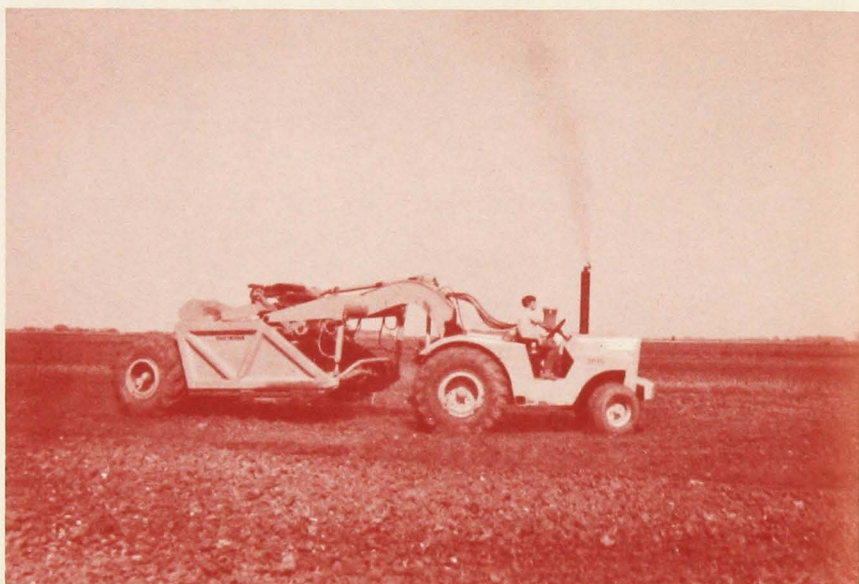
Custom operators are available for land forming.
