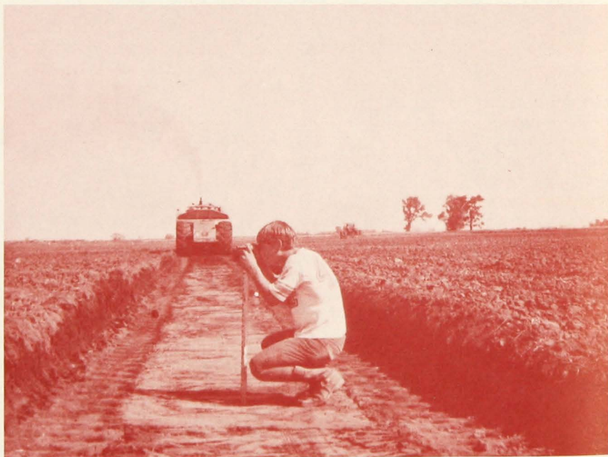
Checking the grade on a land forming project.
