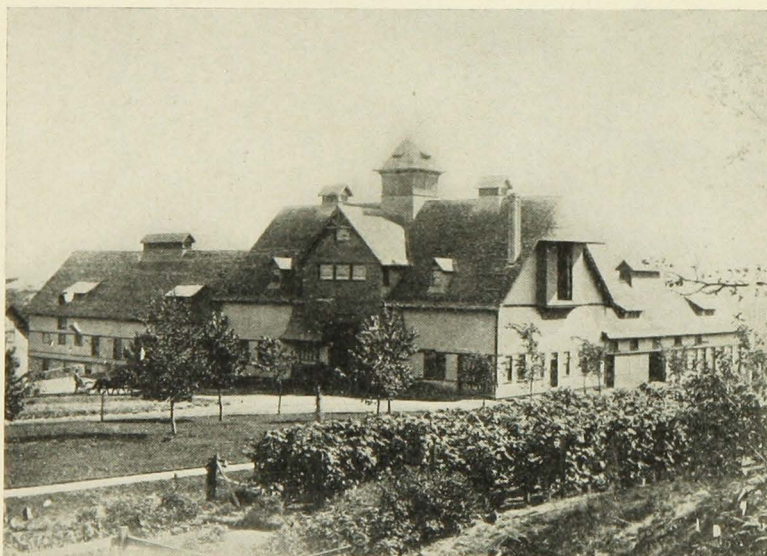
Original Cattle Barn, Experiment Station
