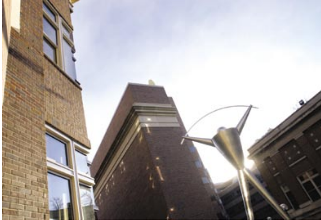
New mechanical engineering facilities—funded in part by campaign contributions—opened in 2001.
