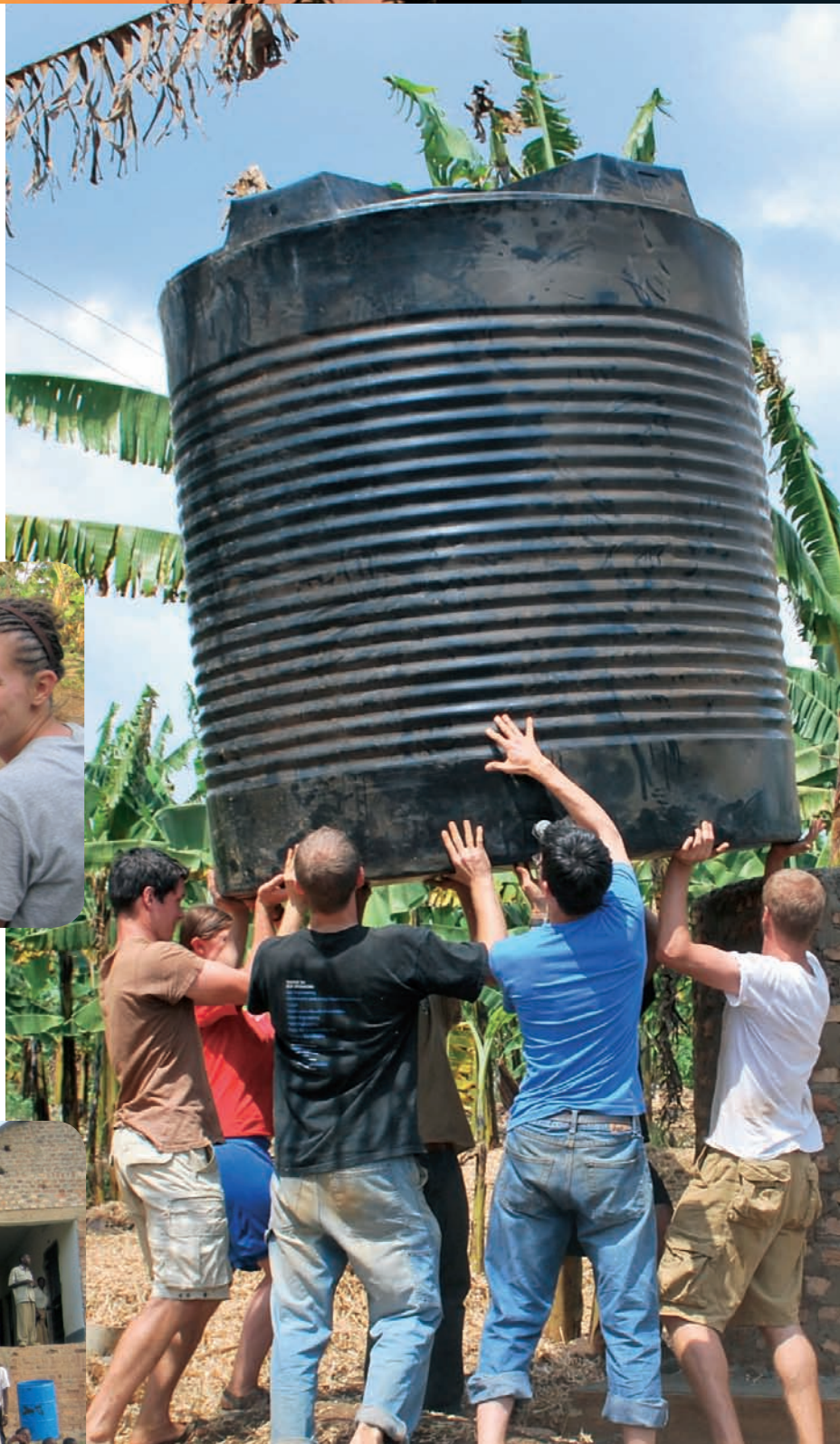
Lifting the 5,000 liter groundwater storage tank into place is (left to right) Scott Andrews, a URF volunteer, Emily Hoskins, Nick Haupt, Nathan Cantley, and Steve Hankey. The tank was placed on an elevated masonry pad that was constructed by a local mason in about three days.
