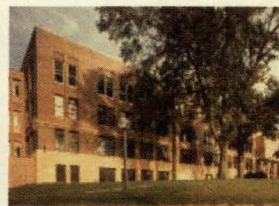
Snyder Hall Addition
