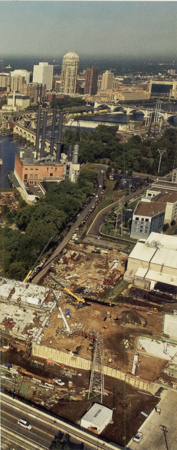
Photographed in mid-August, the new Interstate-35W bridge is about a month from completion. The bridge is 1,223 feet long and has 12 support columns, each 70 feet high. Its 10 lanes opened to traffic on September 18.
