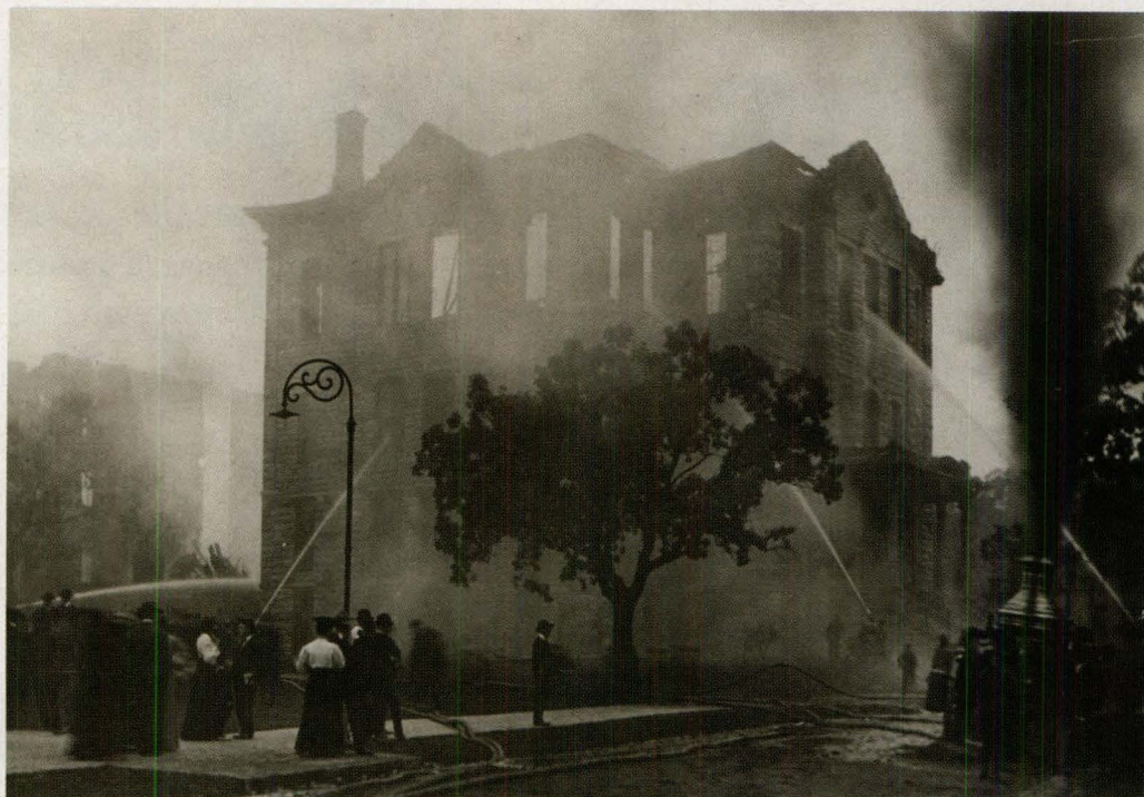
The victim of fire more than once, Old Main burned beyond repair in 1904.
