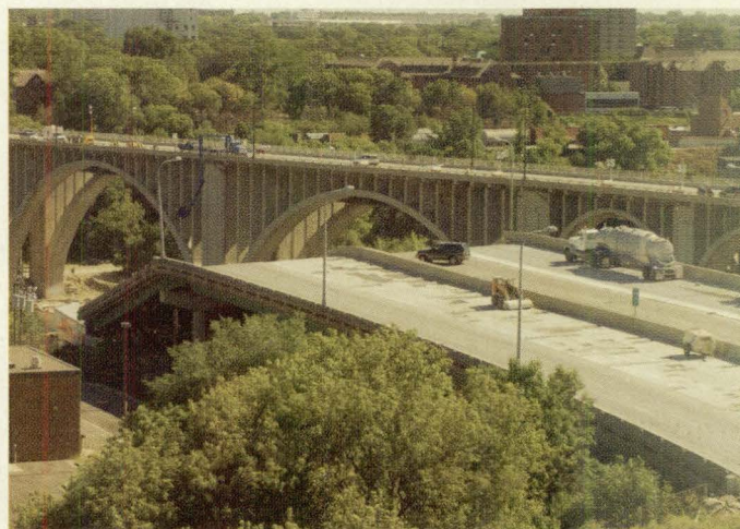
The collapsed Interstate 35W bridge over the Mississippi River as seen from the sixth floor of the University of Minnesota's West Bank Office Building. In the background are the 10th Avenue Bridge and buildings on the U's East Bank campus.
