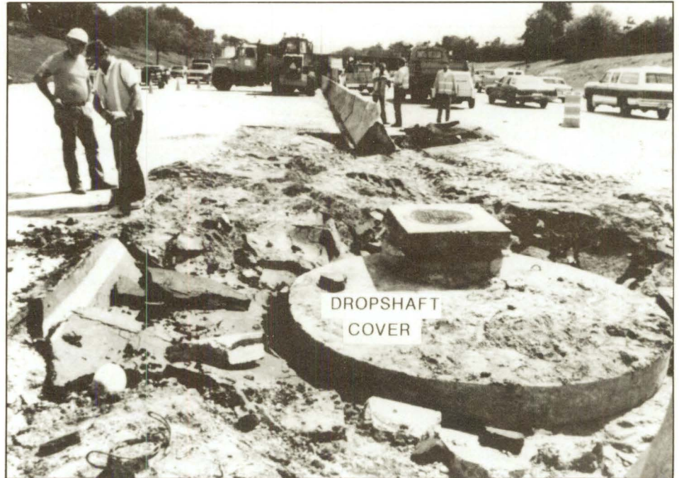
Tremendous pressure builds when storm runoff plunges toward the main sewer interceptors, sometimes literally blowing the cover off dropshafts.
