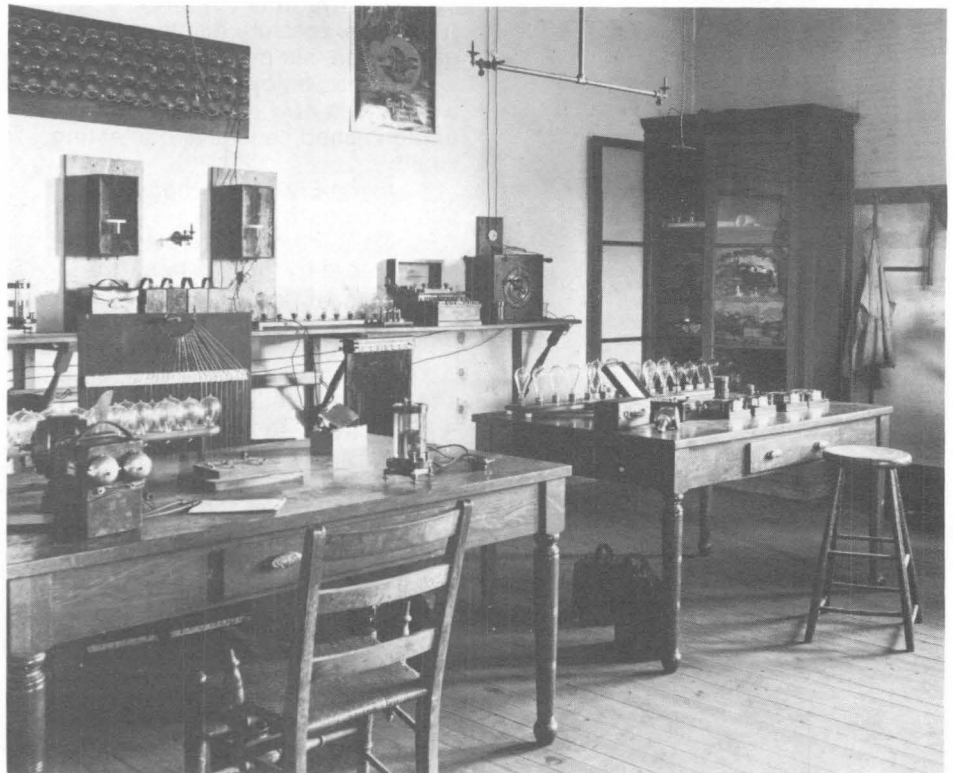
Electrical engineering laboratory in Eddy Hall about the time Ely was a student.
