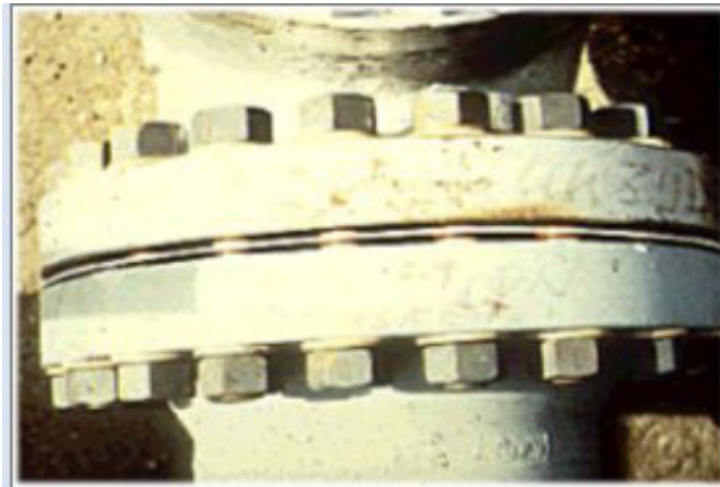
Figure 7: Example of Crevice Corrosion [8]
