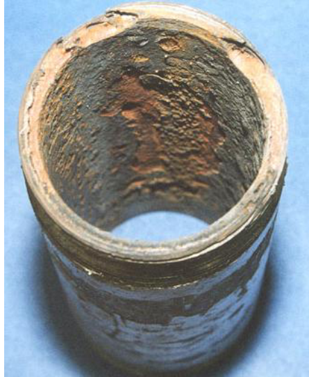
Figure 3: Example of Pitting Corrosion [7]
