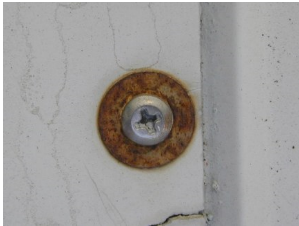
Figure 2: Example of Galvanic Corrosion [7]
