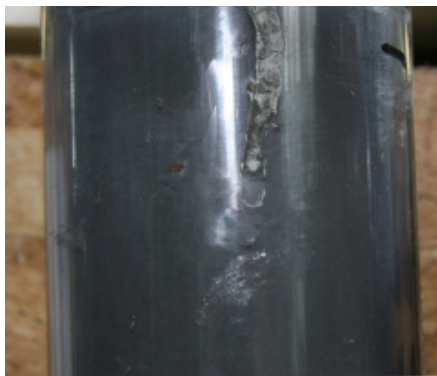
Figure 5: Specimen R-H-1.0-11.5-A, Stain and cracks surrounding stain
