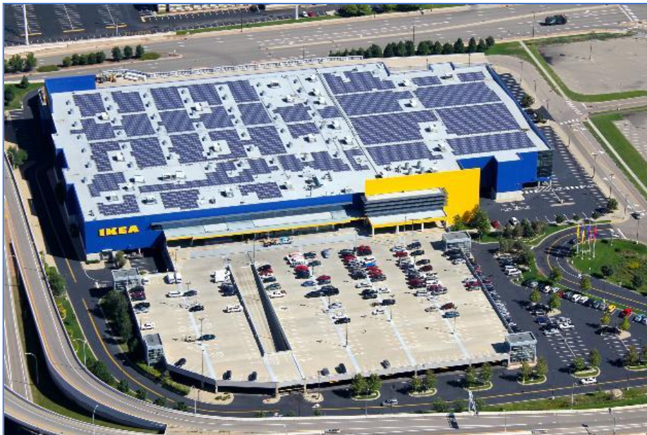
Figure 4. Solar panels on the roof of IKEA in Bloomington, Minnesota. Source: inhabitat.com
