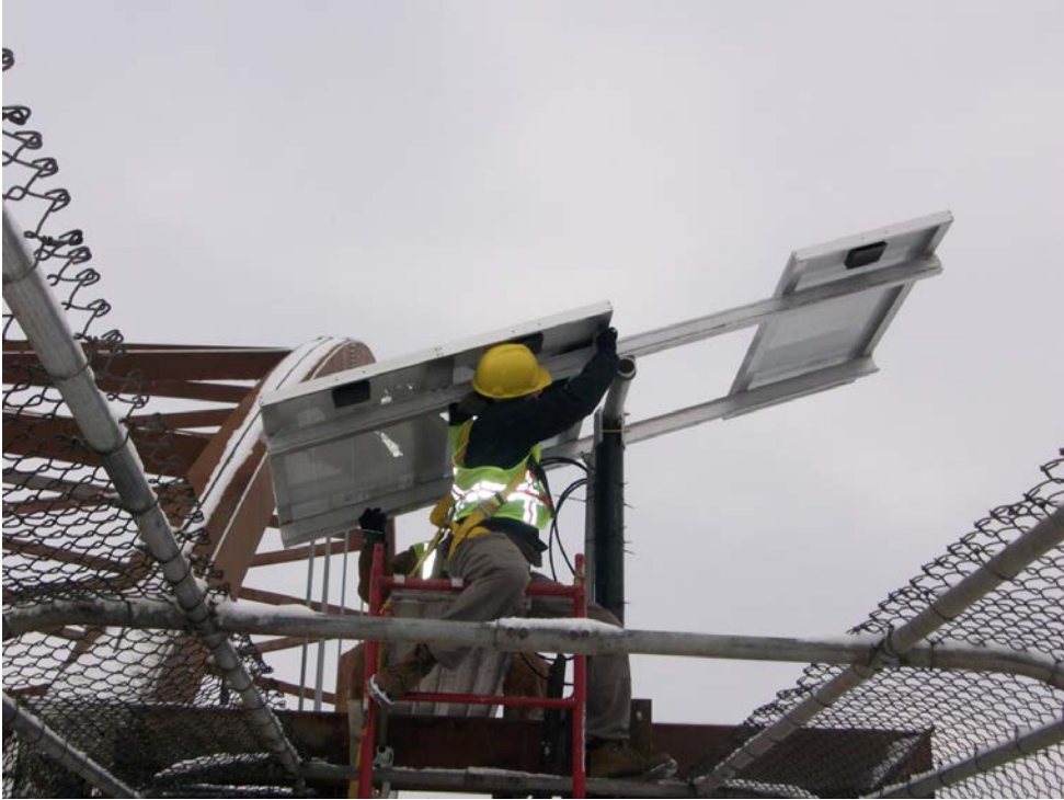
Figure 3.6: Photograph of solar panel installation
