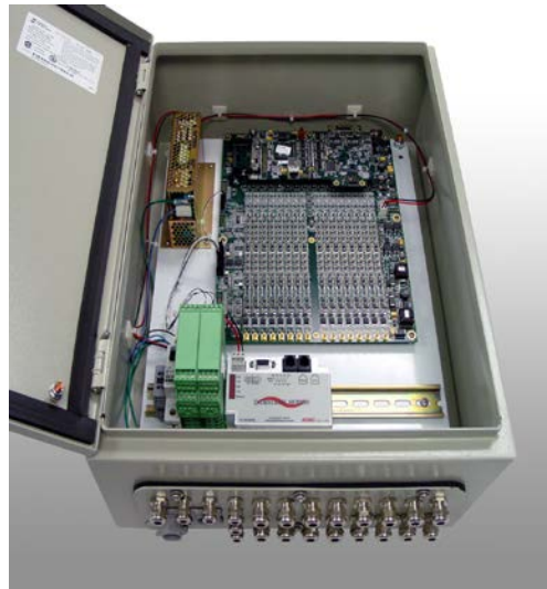
Figure 3.1: Sensor Highway II system (courtesy of Mistras Group, Inc.)
