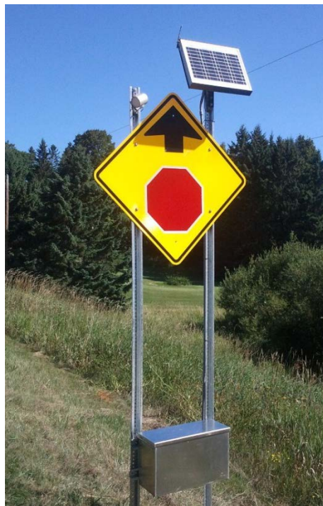
Figure 50: Installed Doppler radar unit (D5) on the minor road.
