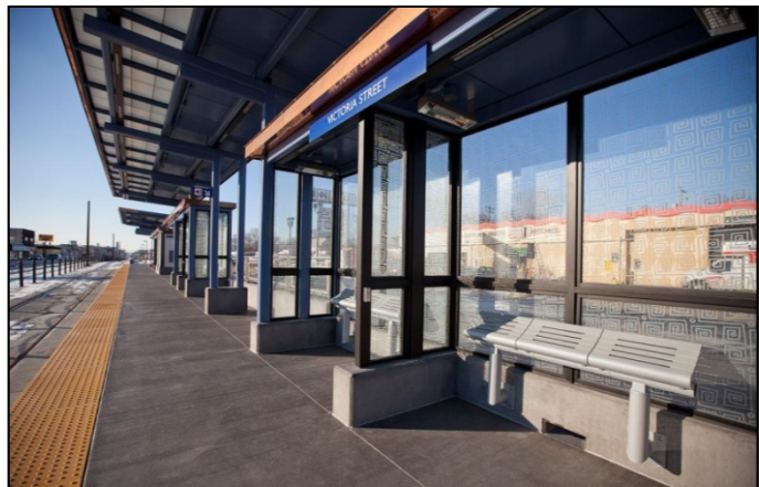
Photo 21: The Green Line Light Rail Station on Victoria Street
