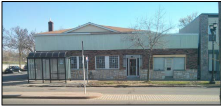
Photo 4: Lack of Curb Appeal
