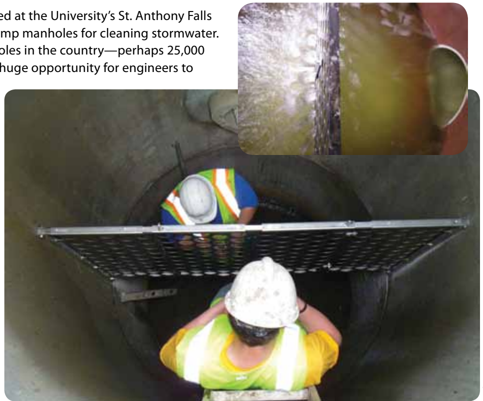
The SAFL Baffle helps keeps sediment and pollutants out of our lakes and rivers.
