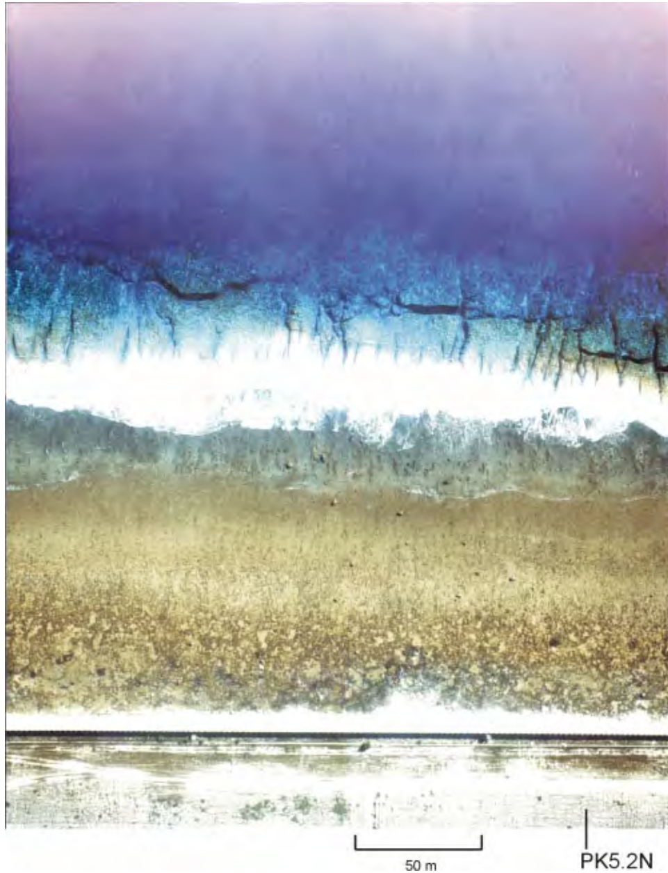
Figure 1.14 Aerial photograph showing underwater extension fractures of the order of 2-m width in the vicinity of PK5N, Irène section (see also Fig. 5.6); part of the aircraft runway strip, with protective wall, runs parallel to the bottom of the photograph; this region is outside test area 1 [photo courtesy of DIRCEN/CEA]
