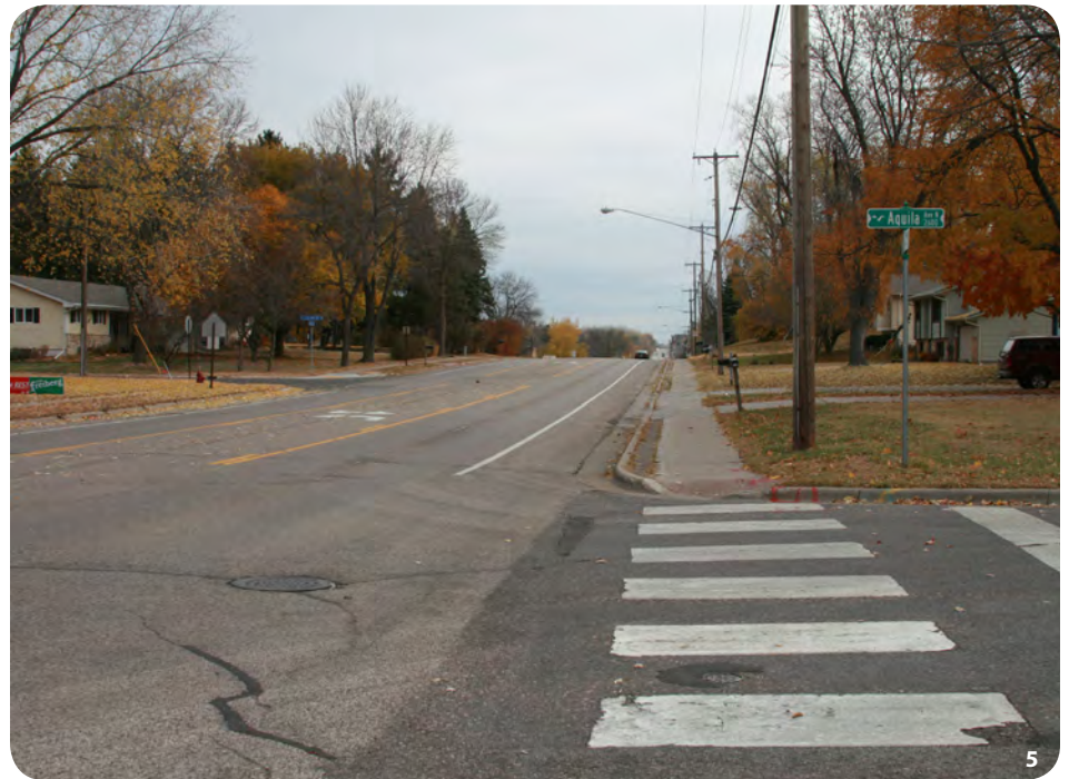
5. This section of Medicine Lake Road was recently converted from four vehicular travel lanes to two lanes and a shared center turn lane. This conversion allowed for the inclusion of bike lanes along this county road.
