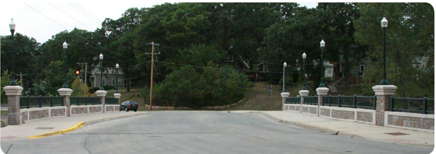
A newly renovated bridge on Lakeview Boulevard in Albert Lea provides wider sidewalks and ramps that are designed to be ADA Compliant.
