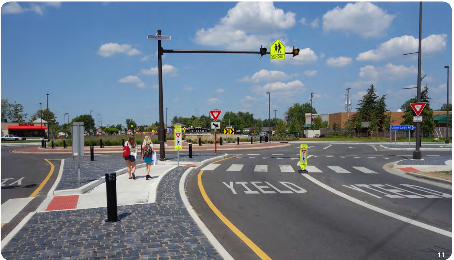
11. The double roundabout was designed to manage roadway traffic, pedestrian and bus traffic from a nearby school, and business access. The roundabout features automobile and pedestrian signage, pedestrian crossings and refuges, roadway and crosswalk striping and pavers, and landscaped center islands.
