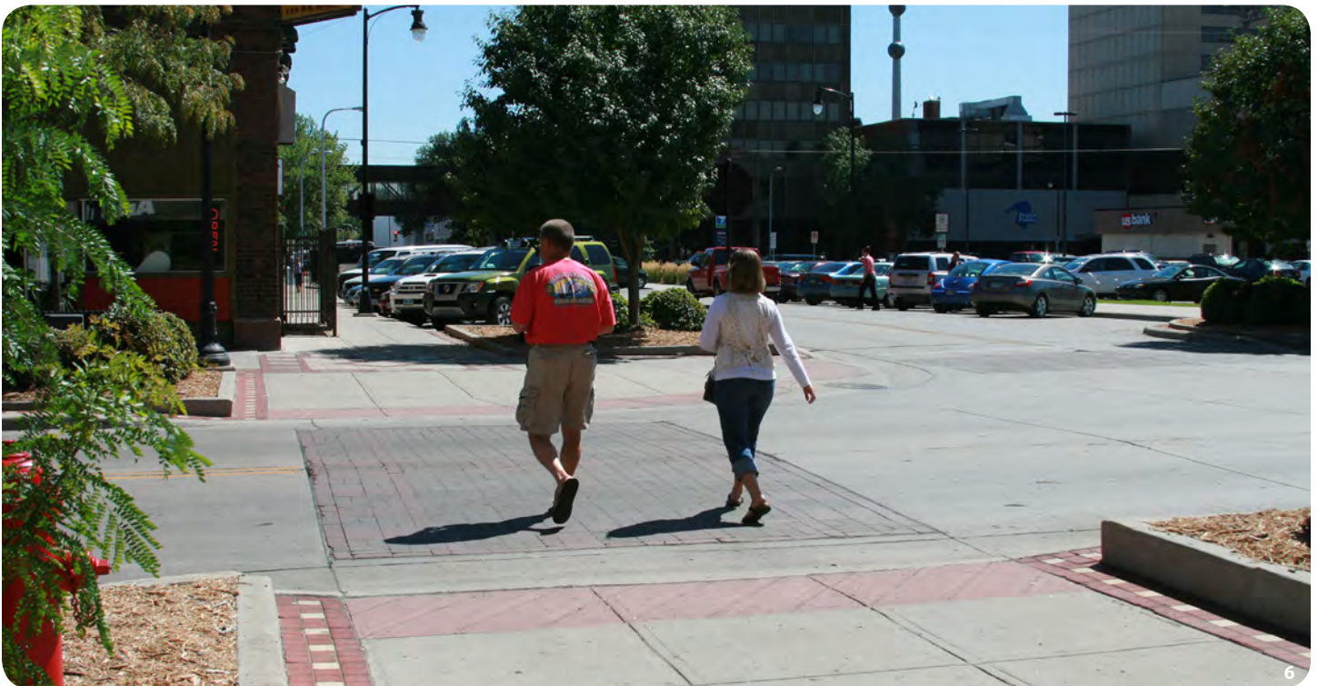
6. Broadway Drive features at grade pedestrian crossings and a change in pavement material clearly delineating pedestrian crosswalks.
