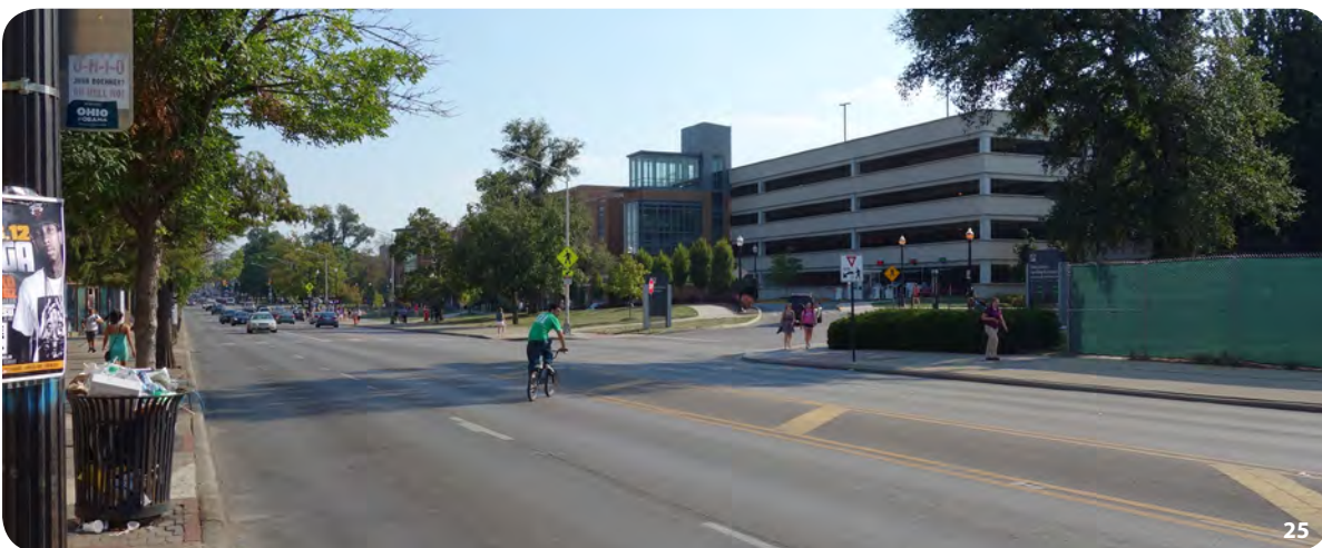
22-25. High Street adjacent to the Ohio State University campus in Columbus, accommodates a high volume of vehicle, transit, pedestrian, and bicycle traffic. Signage, wide crosswalks, and lighted intersections are provided to manage the intersection of modes.
