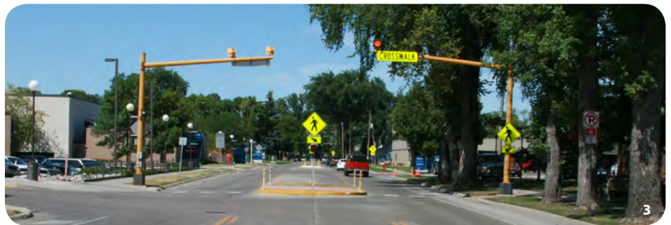
3. 4th Street North in Fargo transects various conditions from urban to residential areas north of the City. Near a medical facility lighted pedestrian signage and a median refuge provide a safe crossing for pedestrians who park across the street and are accessing the hospital, clinic, or pharmacy.
