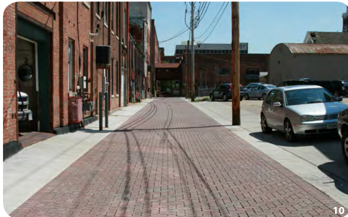
10. Numerous alleys in the Millwork District were also addressed with permeable pavers.
