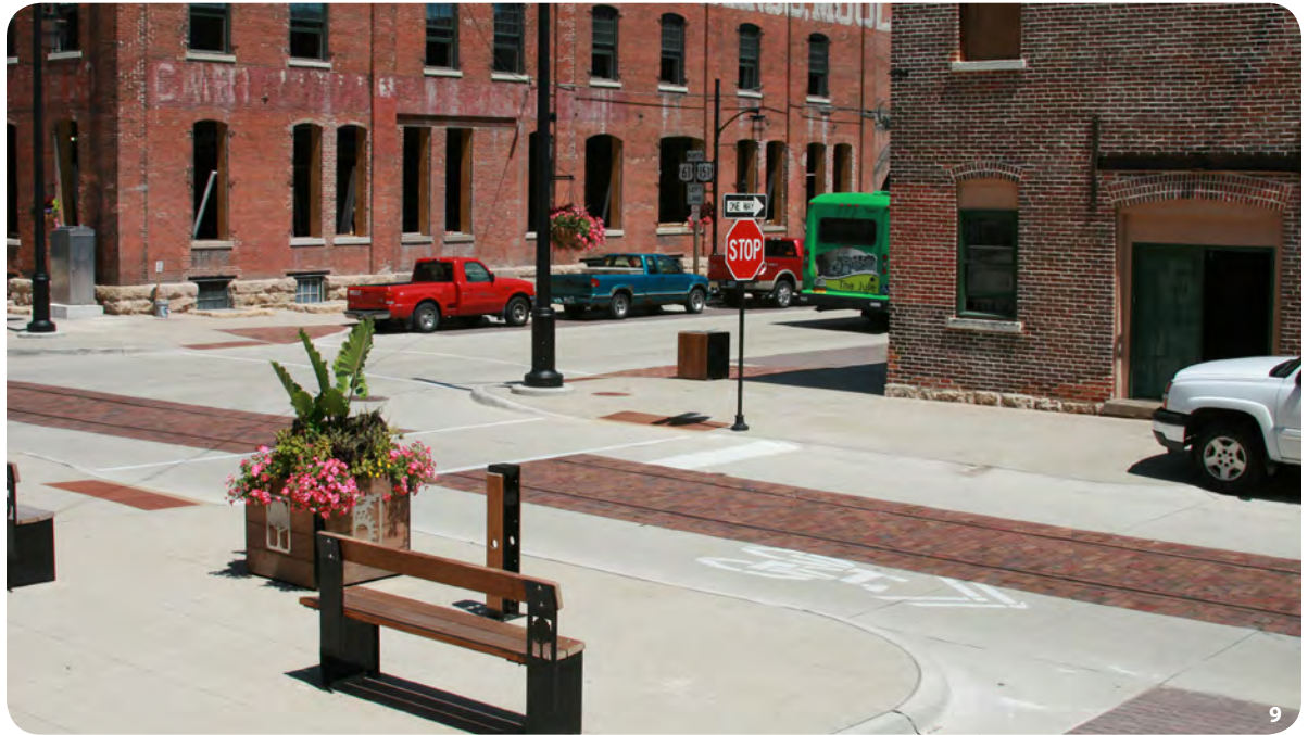
9. The corner of 9th Street and Jackson Street, in the heart of the Millwork District, incorporates historic details, new seating, planters, bike racks, and ample room for pedestrians.
