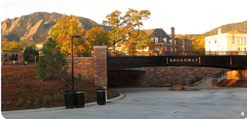
6. A new underpass under Broadway Avenue connecting the University of Colorado Boulder and an adjacent neighborhood provides pedestrian and bicycle access on one of the city's busiest arterials. The project brought together funding from multiple sources including the University. Source: downclimb flickr stream
