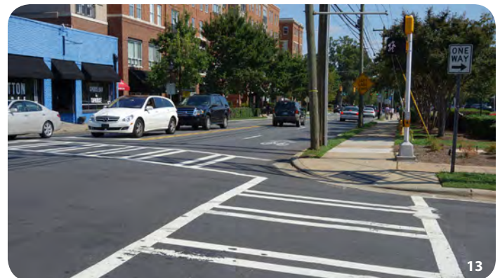
13. East Boulevard and Kenilworth Avenue intersection in the Dilworth neighborhood. Existing development along the roadway offers limited right-of-way and thus a combination of bike lanes and sharrows are used to accommodate bicycles on this busy commercial street. Enhanced crosswalks and pedestrian signals are also provided.
