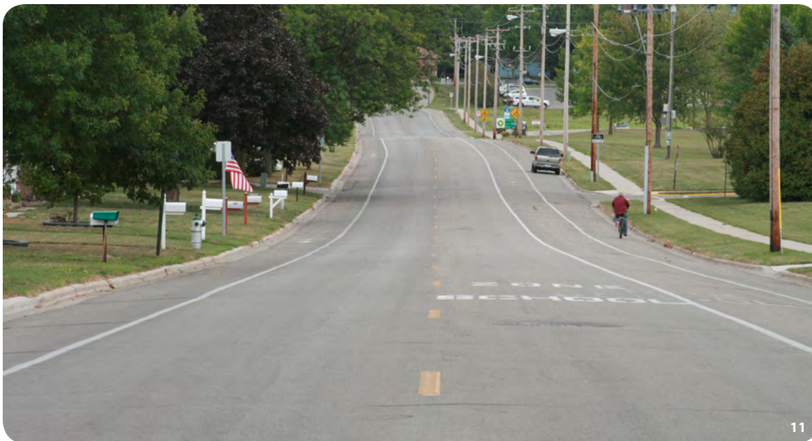
11. The City's first bike lanes were implemented on Front Street, a major arterial that transects many different conditions in Albert Lea. In this section in front of an elementary school, parking was removed on the side of the street across from the school to allow for wide bike lanes and the school zone is marked to increase safety for students.
