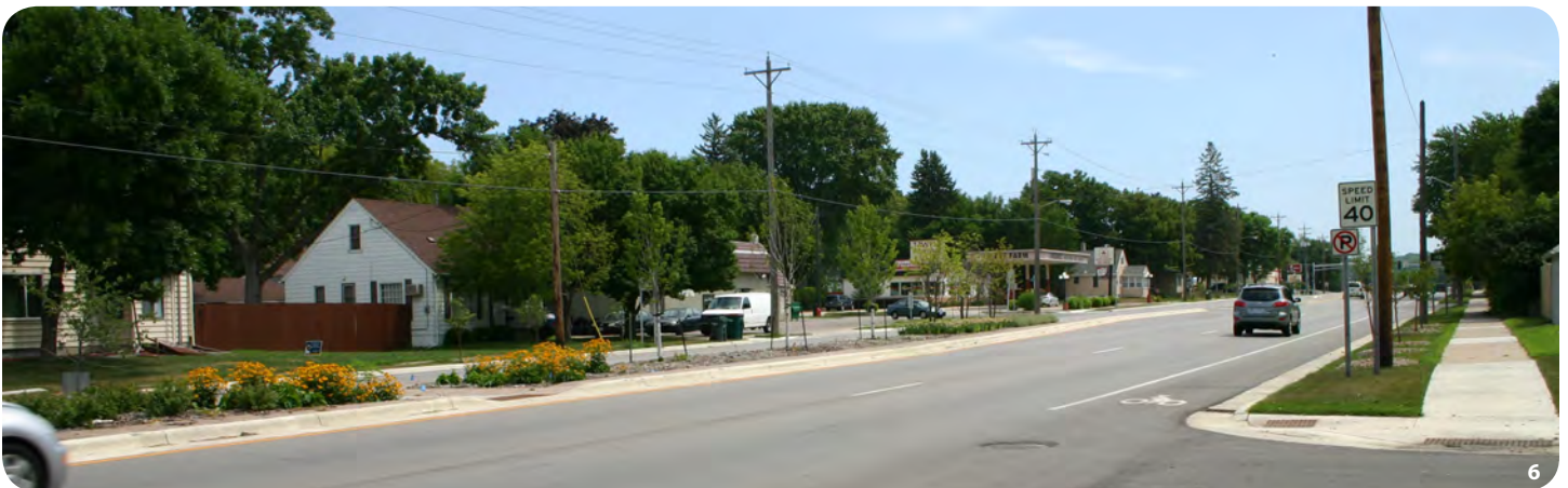
6. 12th Street in southern Rochester was recently reconstructed and the City implemented medians with pedestrian crossings, a bike lane, and ADA compliant ramps in the redesign of this busy corridor.
