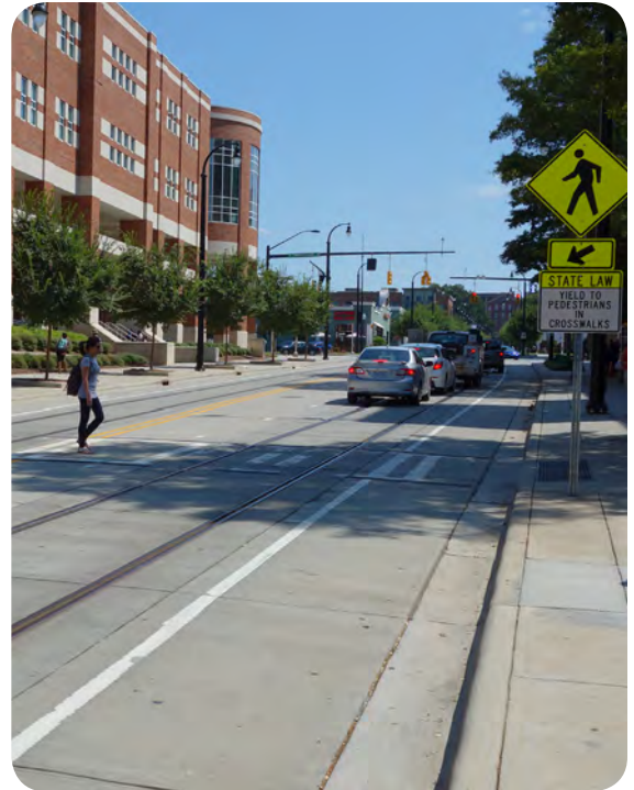
On a new campus of the Central Piedmont Community College near downtown Charlotte, streetcar tracks have been installed in anticipation of future rail service.
