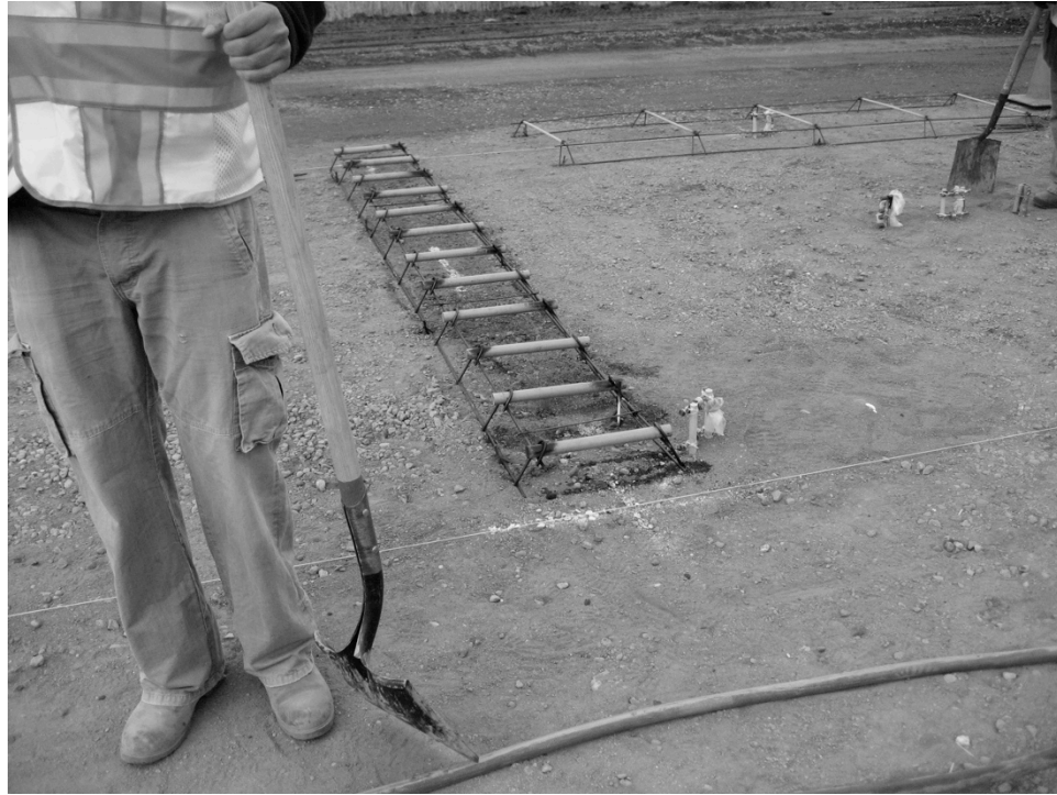
Figure 2.3 Dowel bars in baskets placed on JPCP base layer prior to placing the concrete layer
