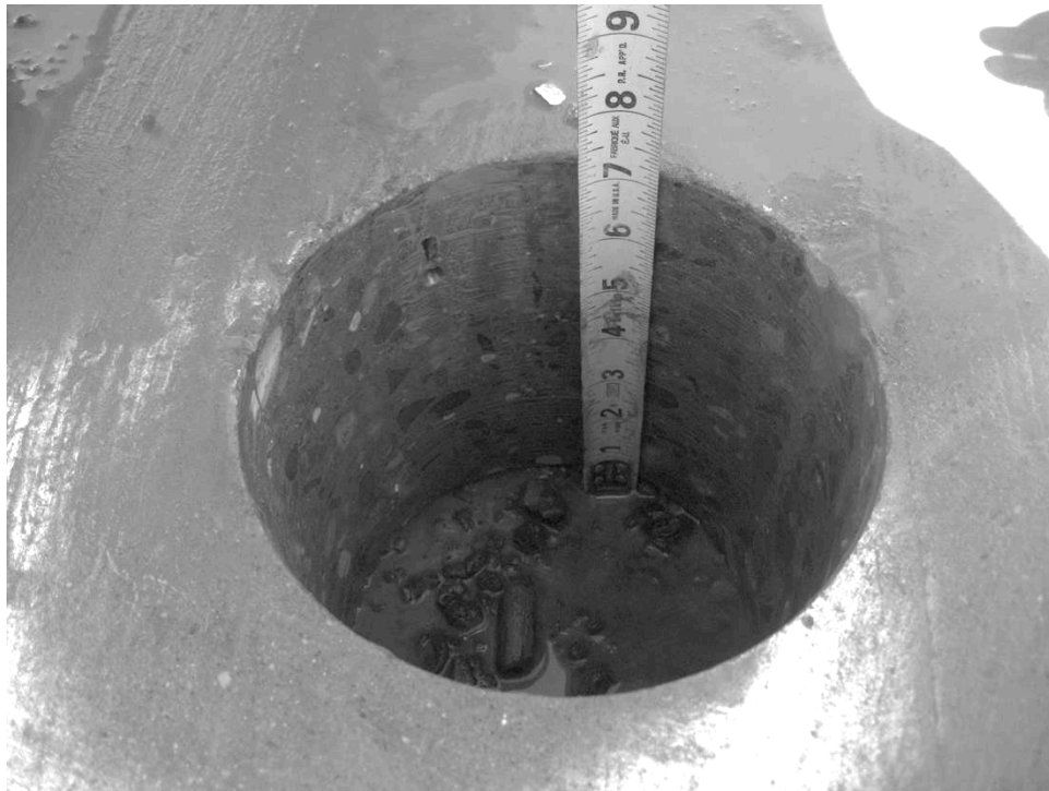
Figure 2.4 Hole resulting from drilling a concrete core for thickness measurements
