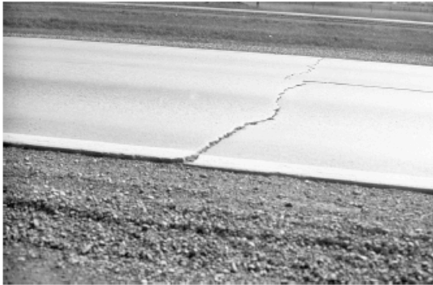
Figure 2.6 Example of a JPCP transverse crack
