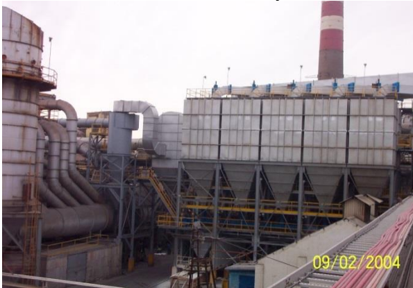
Filtration Equipment: House of Bags increasing the filtration capacity to more than 3.5 million m 3 /Hour.
