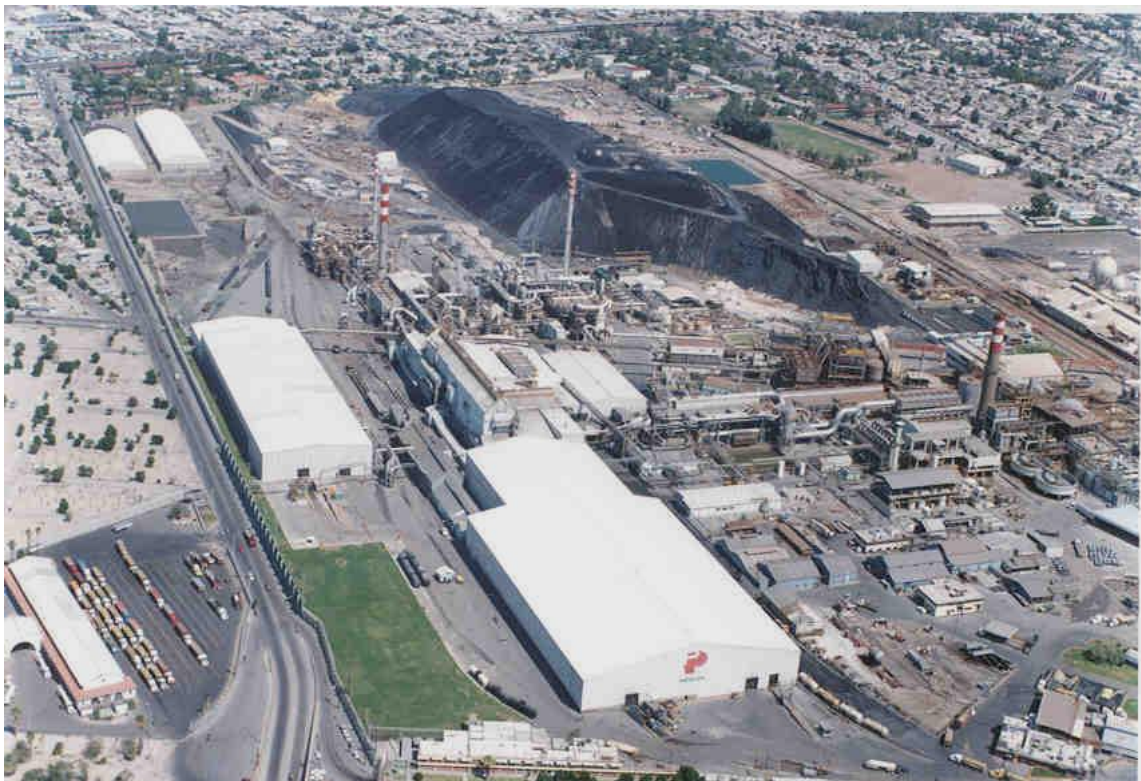
Figure # 5: Aerial Photo of the Smelter: Development of warehouses: > 45,000 \text{m}^3 were built keep all processes of lead production encapsulated to prevent fugitive emissions of lead particles to the atmosphere, keeping air emissions under control.
