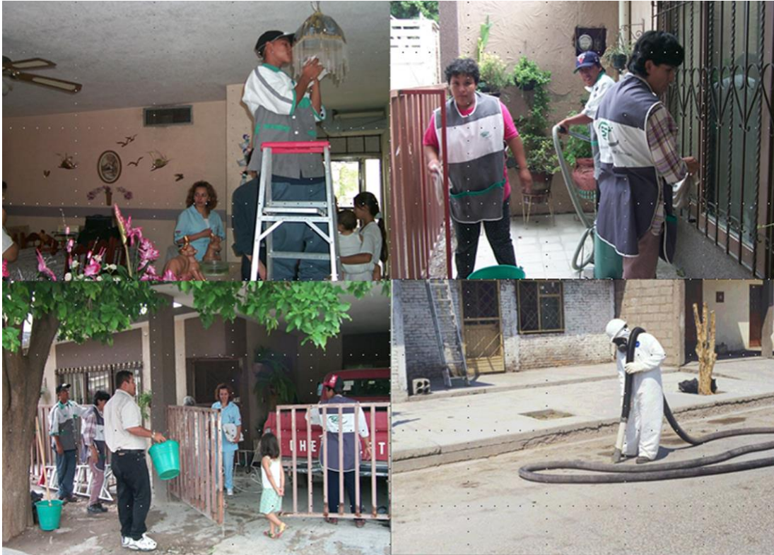
Figure # 14.- Indoor Environmental Remediation: A large number of people from these communities received training on lead hazards & decontamination then were hired to work full-time performing environmental cleanup and remediation of households: Thorough cleaning inside houses by wet-cleaning methods, vacuuming indoors to include windows and door edges, all furniture, floors, roofs and all exterior structures of each house. Indoor cleanup remediation was performed periodically at each household until Blood Lead Levels from household children with high Blood Lead Levels fell off below 10 \mu\text{g}/\text{l} .
