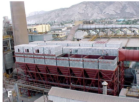
Figure # 6: Control of air emissions: New Technology implemented to control all emissions of lead from the smelter by making structural and technology changes. A: Warehouse to Process Zinc Concentrates, B: Warehouses to Process Secondary Processes, C: New Filtration Equipment at Cold Sintering Area, D: Modern Electrostatic Precipitator, E: Increasing the House of Bags to capture particles and F: House of Bags. All filtration systems filter more than 3 million 3m per hour.
