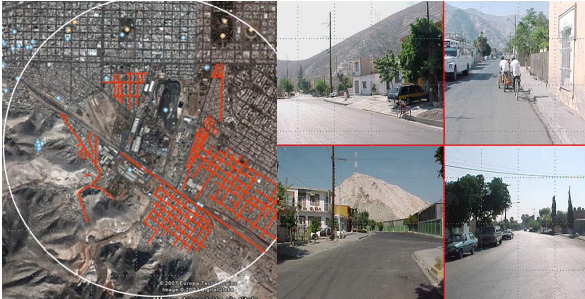
Figure # 12.- Pavement of the Streets and Roads: Aerial Figure # and Streets around the smelter. More than 400,00 m 2 of pavement were placed on unpaved roads and streets around the smelter. These included the pavement on the following neighborhoods (Colonias) E. Guerra 155,021 m 2 , 1° de Mayo 19,608 m 2 , V. Guerrero 68,806 m 2 , L. Echeverria 36,032 m 2 , Cañon del Marmol 27, 271 m 2 , , M Aleman 16,429 m 2 & Other Colonias 36,032 m 2 .
