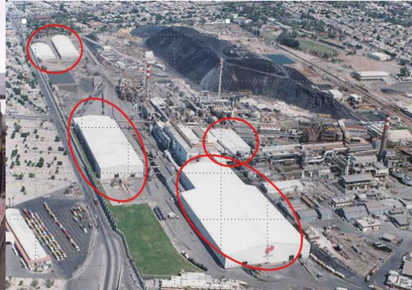
45,000 m 2 Warehouses were built to keep all processes indoors and prevent fugitive lead emissions to the atmosphere
