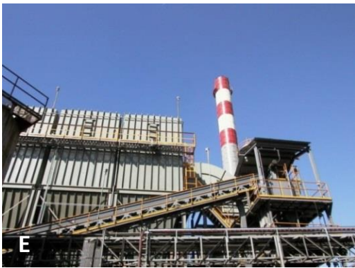
Figure # 6: Control of air emissions: New Technology implemented to control all emissions of lead from the smelter by making structural and technology changes. A: Warehouse to Process Zinc Concentrates, B: Warehouses to Process Secondary Processes, C: New Filtration Equipment at Cold Sintering Area, D: Modern Electrostatic Precipitator, E: Increasing the House of Bags to capture particles and F: House of Bags. All filtration systems filter more than 3 million 3m per hour.
