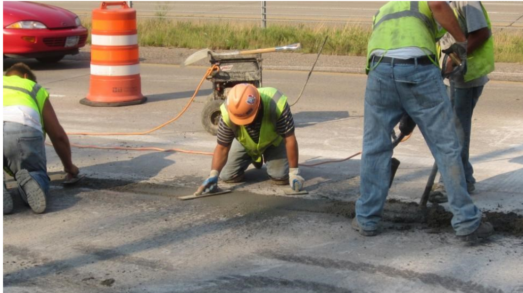
Figure 72: Placement, consolidation and finishing
