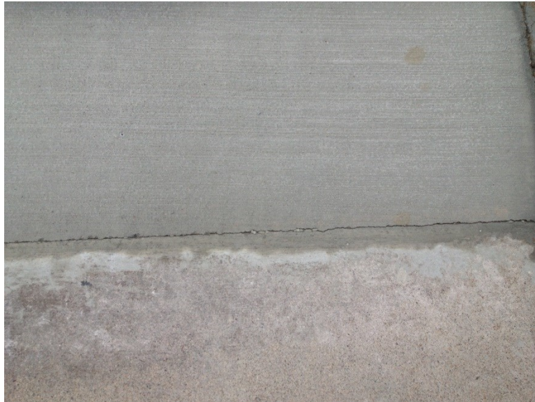
Figure 62: Edge de-bonding due to shrinkage along a saw-cut patch area
