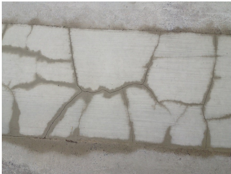
Figure 64: Cracked patch that was placed with no curing
