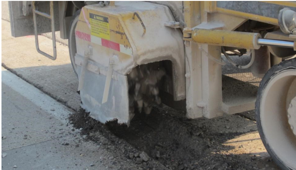
Figure 65: Milling machine grinding a spalled section of concrete
