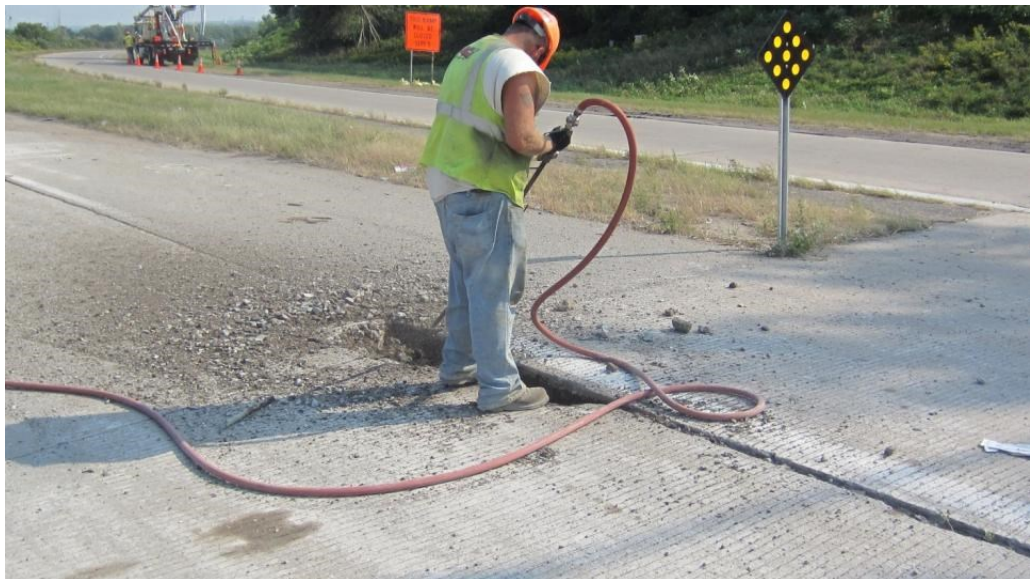
Figure 67: Air blasting the hole to remove excess loose material
