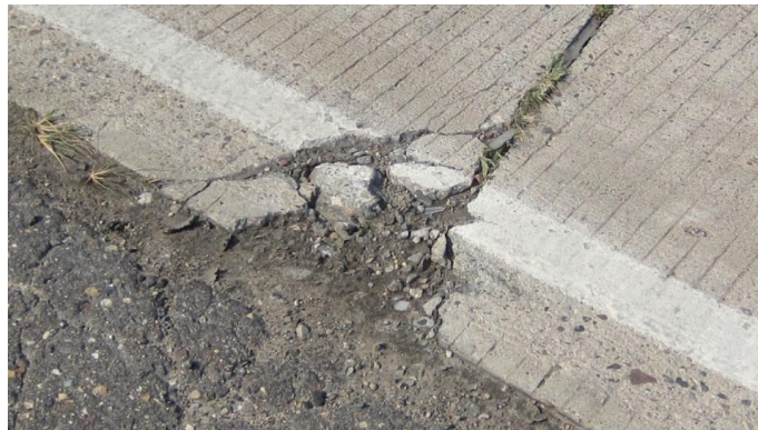
Figure 1: A spall ready for grinding
