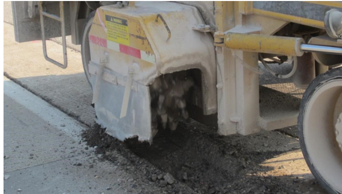
Figure 2: The grinding machine removing material on a spalled section of pavement
