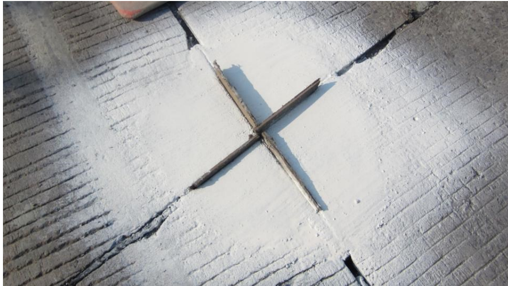
Figure 74: A finished patch with fiber board inserted to maintain a working joint
