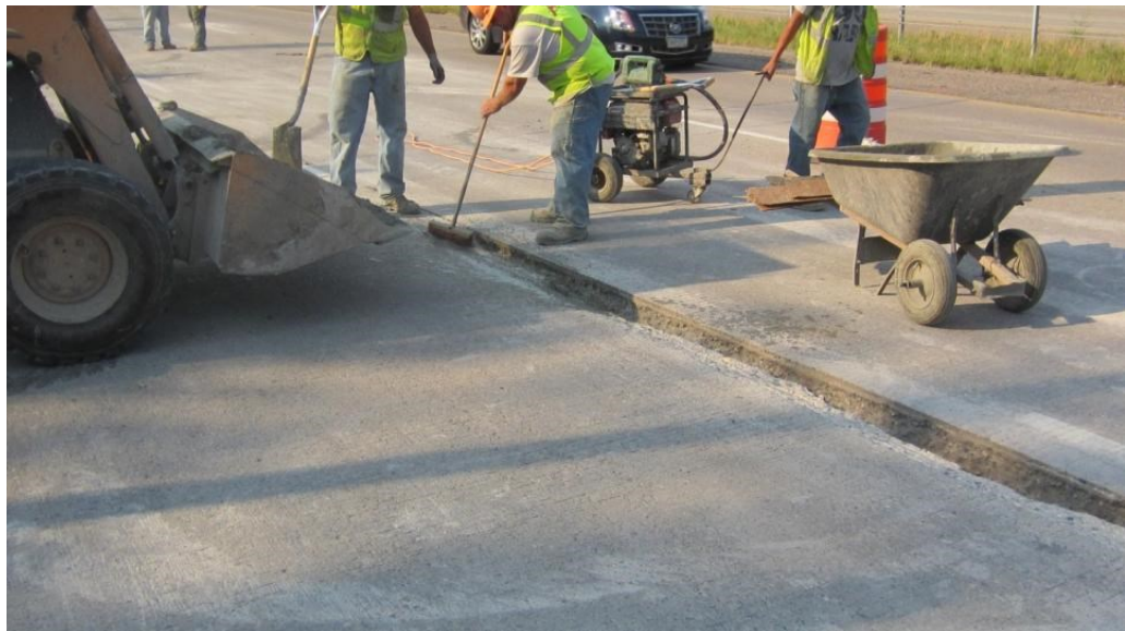
Figure 71: Applying the concrete slurry that provides adhesion for the patch material
