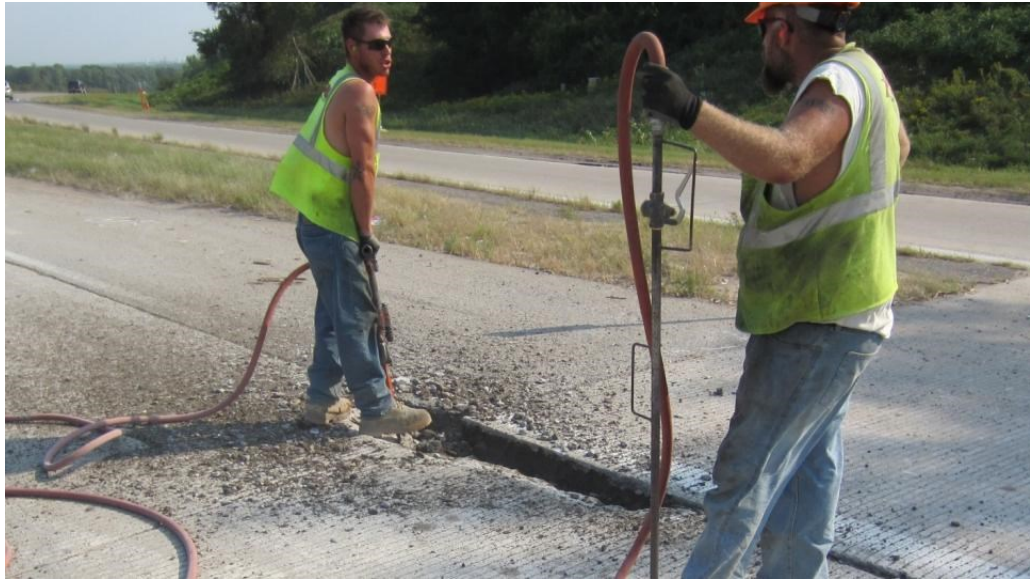
Figure 66: Chipping the edges to meet MnDOT specifications
