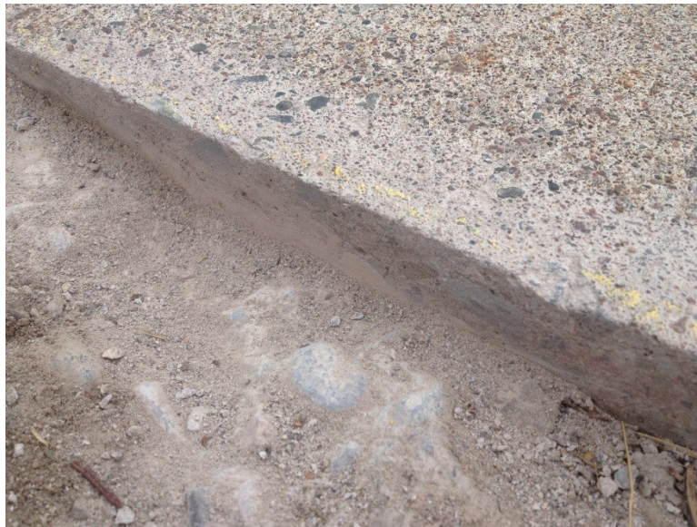
Figure 60: Saw-cut edge of a patch area, vertical face
