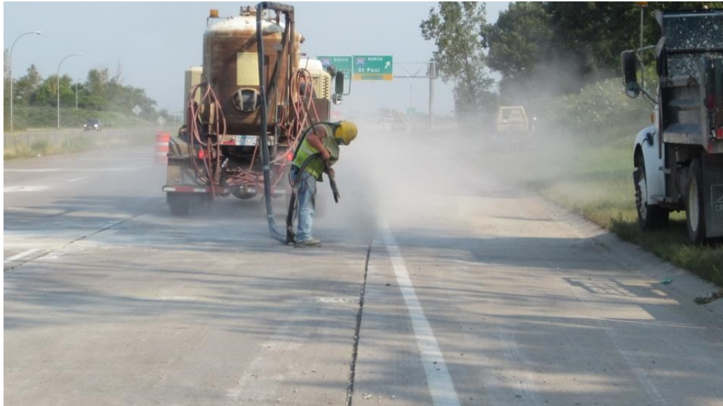
Figure 68: Sandblasting the patch area prior to being filled
