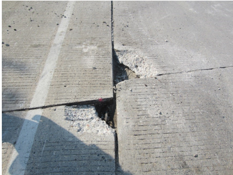
Figure 61: Tapered edges of two opposing corner partial depth repairs
