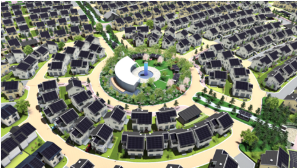
Figure 1.11: The Fujisawa Sustainable Smart Town (FSST) is being built by Panasonic (one of nine Japanese companies participating in the project) on a former industrial site outside of Tokyo. A commercial broadcast in U.S. markets features the design and building of FSST as just one of many green initiatives by Panasonic (above). Despite the circular center of the town, its plan largely follows a suburban single-family housing pattern that will look familiar to American audiences. Upon closer inspection the prominent “black” roofs are revealed to be solar panels (below), the most visible feature denoting its technological systems and connoting its environmental sustainability.
