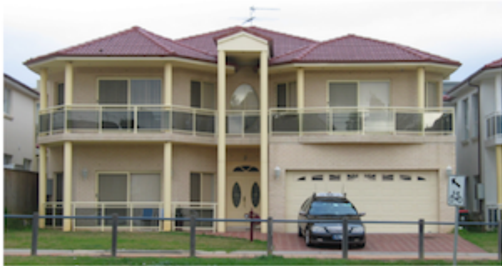
McMansion produces 80 tonnes of CO 2 in construction. Produces 44 tonnes of CO 2 annually
