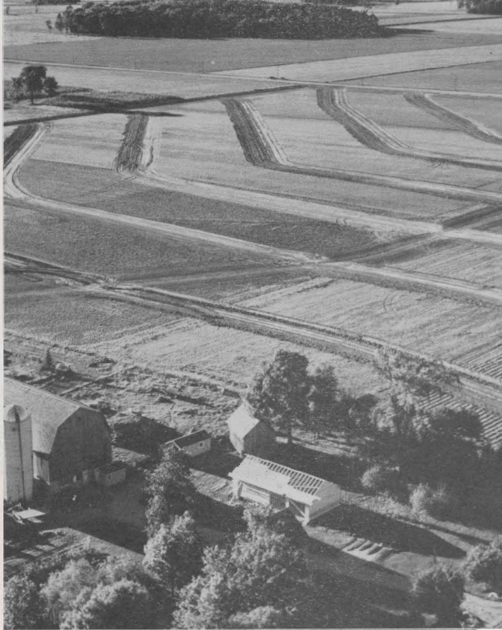
These parallel terraces cover 40 acres. Rows now will run parallel to the terrace rather than up and down hill (as in lower right now). Note outlet waterway, terrace.
