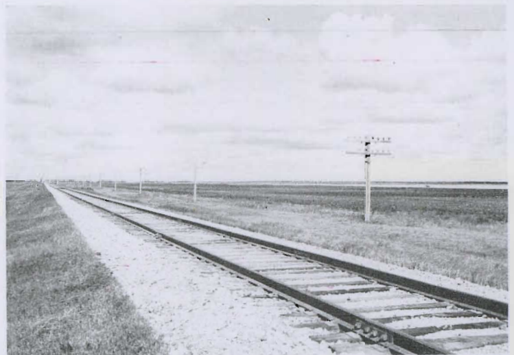
Fig. 2. Notice the level lay of the land in the Red River Valley.
