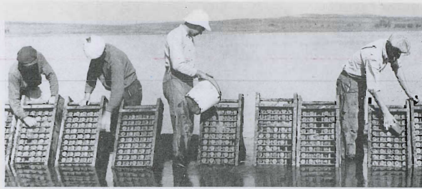
This photograph shows crates of cylinders being prepared for their annual inspection after being exposed to the bitter, sulfate waters of Medicine Lake.
