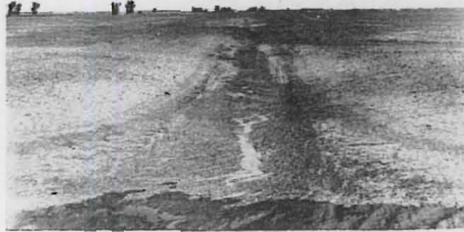
Fig. 4. Type of broad, shallow, straight ditches used to drain Rocksbury soil.
