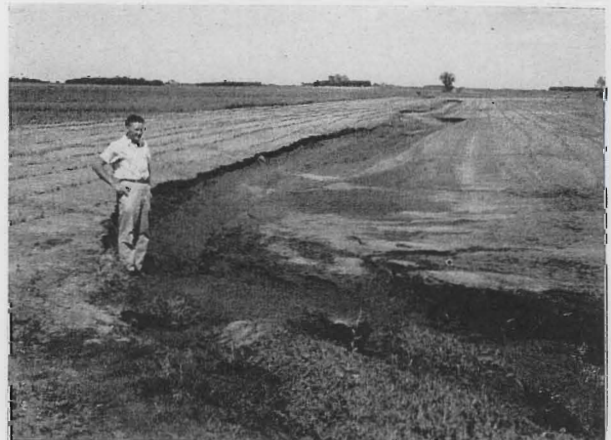
Fig. 2. Erosion resulting from 11-inch rain in a flat waterway which had not been seeded down. Near Clarkfield.
