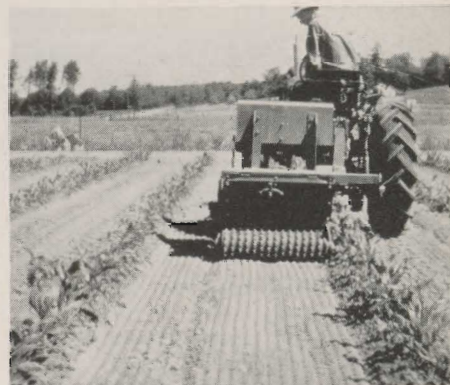
Fig. 6. Roller-seeders which run between the young corn rows are also being used in studies on interseeding. Larger versions of this experimental model have been developed by farm equipment manufacturers.
