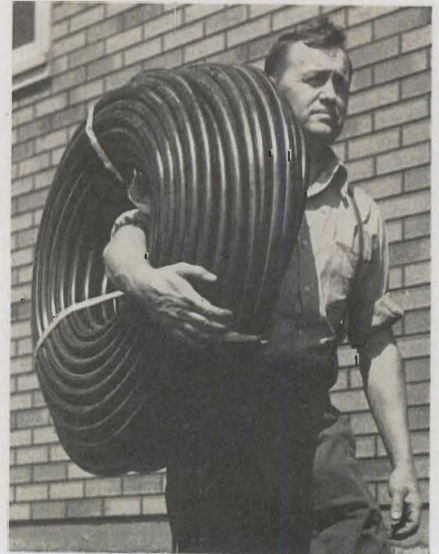
Fig. 2. Workman carrying a 400-foot coil of \frac{3}{4} -inch plastic pipe (approximate weight 56 pounds).
