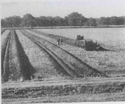
On this flat land near Le Sueur, draining with tile spaced 100 feet apart and 3½ to 4 feet deep made a planned rotation possible.
