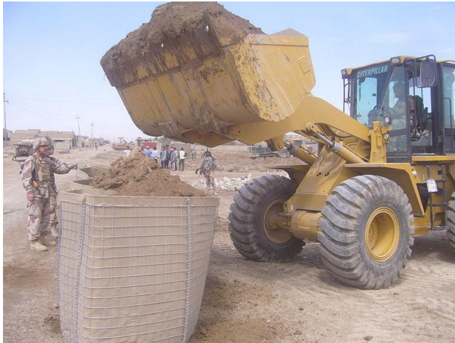
Fig 1-2 Hesco bin being filled w/ front end loader Image: http://xbradtc.wordpress.com , 2008
