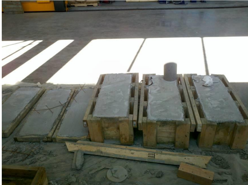
Fig 3-6 Concrete box sections and lids in forms
