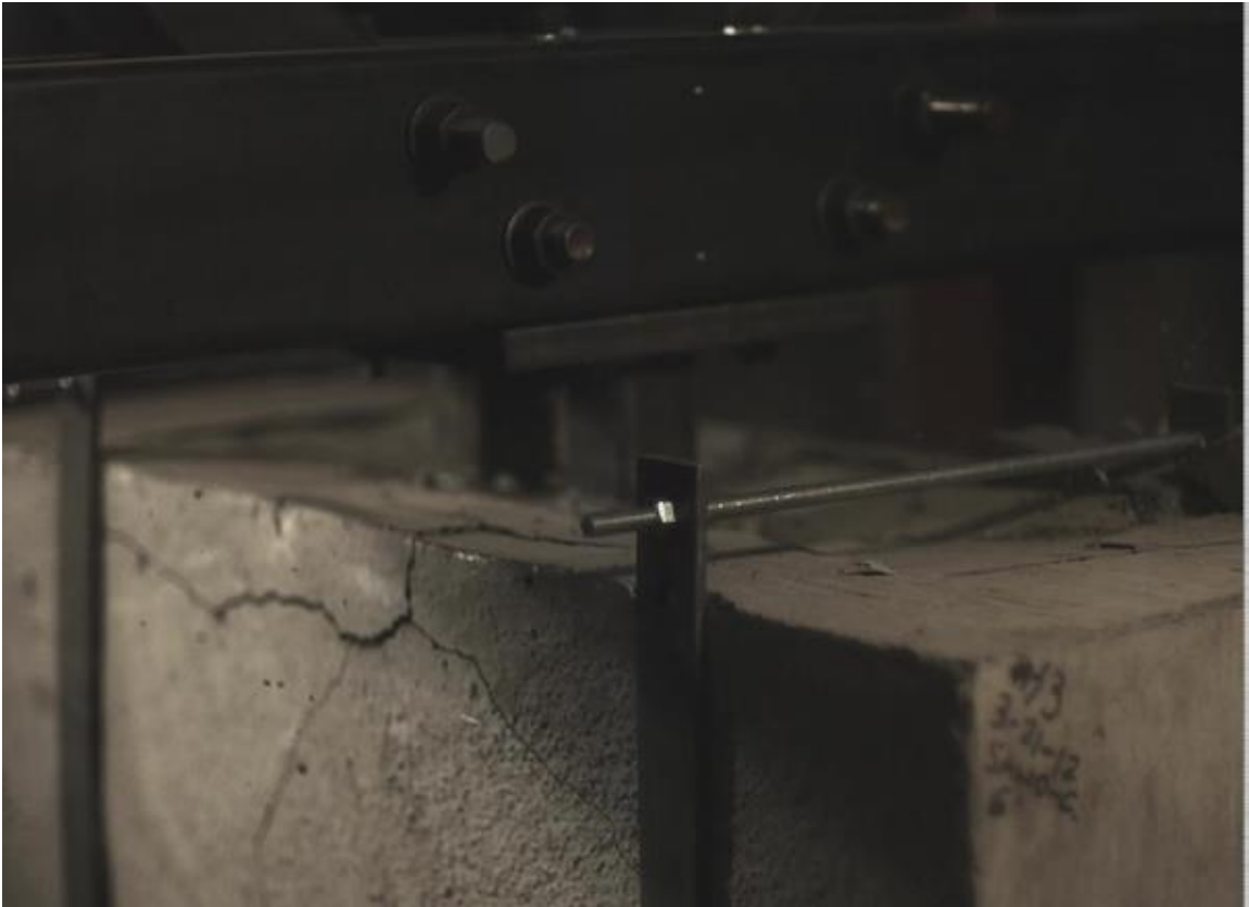
Fig 4-49.1 Test 13 – Plate Sand Compacted Bottom cracking
