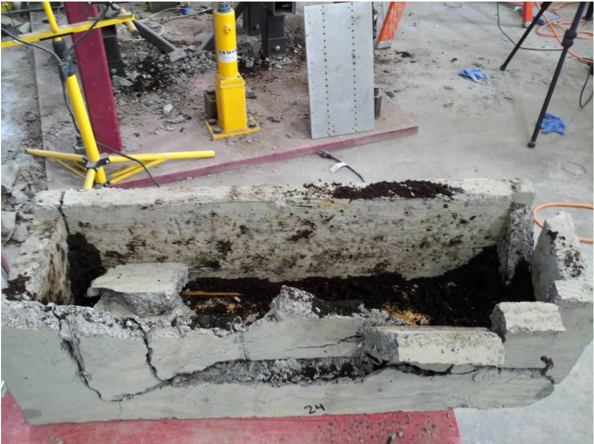
Fig 4-59 Test 24 – Plate Soil Compacted II Emptied
