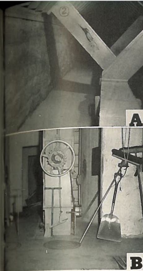
Fig. 13. A. Conveyor tunnel in an elevator showing cemented floor and plastered rock walls, thus eliminating insect harborages and facilitating cleaning. B. View of the work floor of a modern concrete country or line elevator where good housekeeping is a routine practice.
