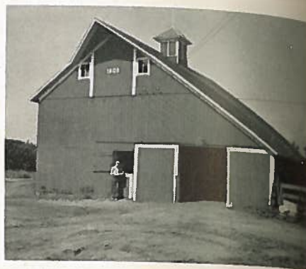
Fig. 8. A combined livestock barn, hay barn, and granary. Such structures prevent the natural, seasonal cooling of grain stored in them, and permit activity of stored grain insects throughout most of the year.
