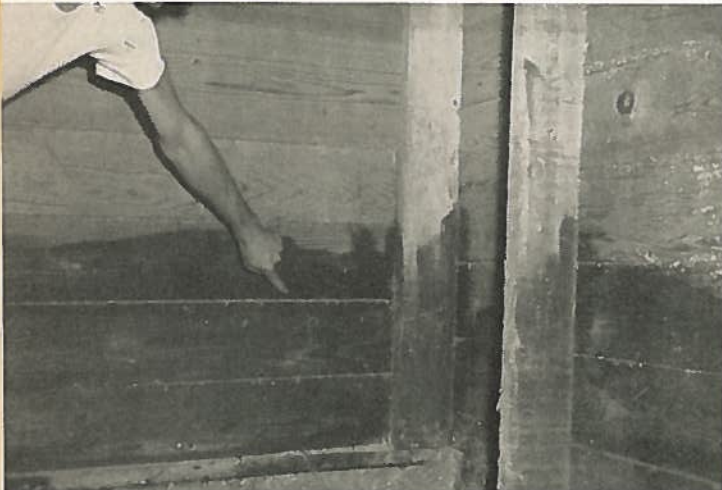
Fig. 3. A corner of a wooden bin showing the accumulation of grain in the cracks between the wallboards and on the floor.
