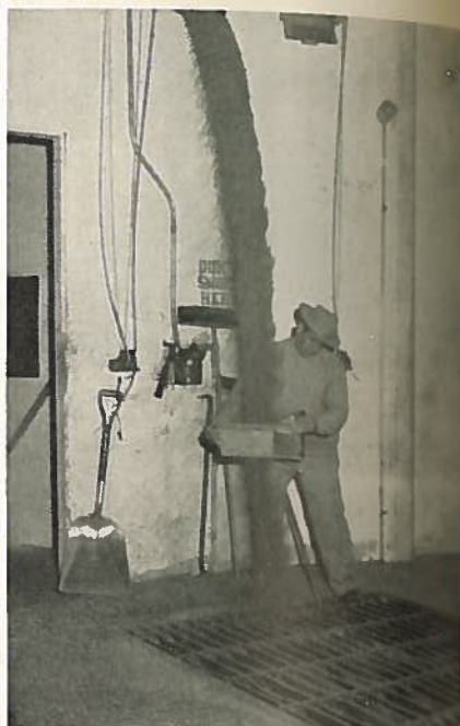
Fig. 14. Sampling elevator grain with a pelican sampler.
