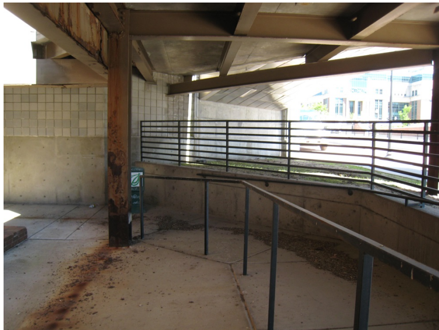
Stairwell at transition between street level and approach up stairs to Washington Ave pedestrian crossing. Undesirable walking environment with concentrated bird roosting overhead. Difficult conditions to create ADA compliant access.
