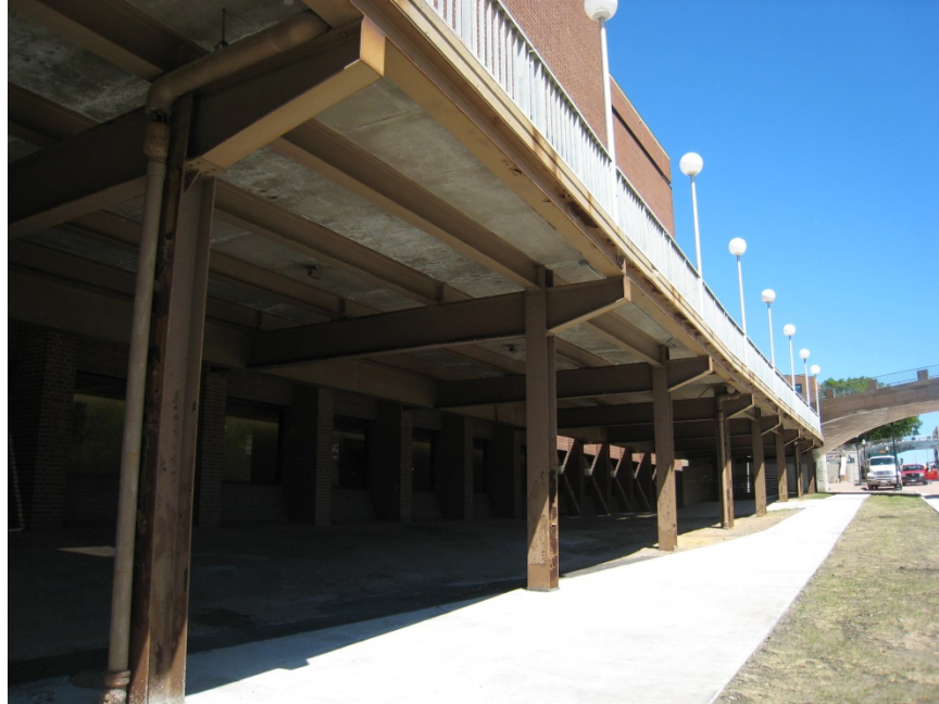
Deck creates perception of lurking space and unpleasant walk environment for pedestrian traffic moving along sidewalk between Coffman Union/ Northrop Mall transit stop and STSS building at Washington Avenue bridgehead.
