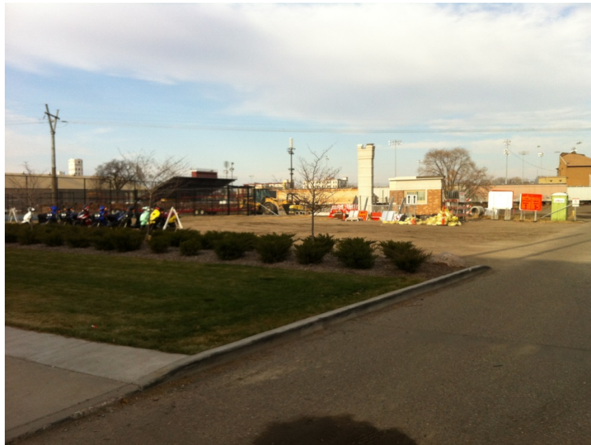
Present day view of site from 5th Street. Facility would be located behind tennis courts (location of parked excavator.)
