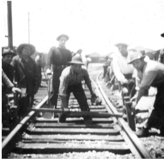
Figure 3.3 Railroad guest workers repairing track on the Southern Pacific Railroad line, Oakland, California, in 1944. Photographer unknown. Personal photograph. Source: Collection of Oakland Museum of California. Gift of Jose Cruz. http://www.museumca.org
