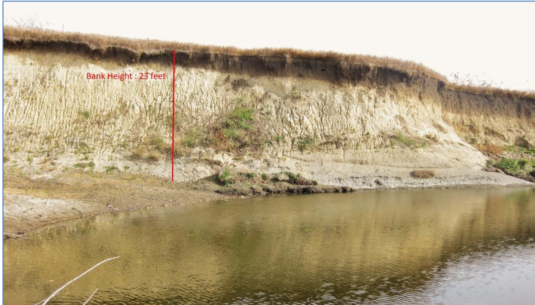
Figure 2.3 Actively eroding streambank on Elm Creek, a tributary to the BER. Photo by Presnail, taken fall, 2011.
