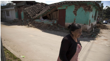
Image: Adobe dwelling affected by earthquake in Guatemala 2012
