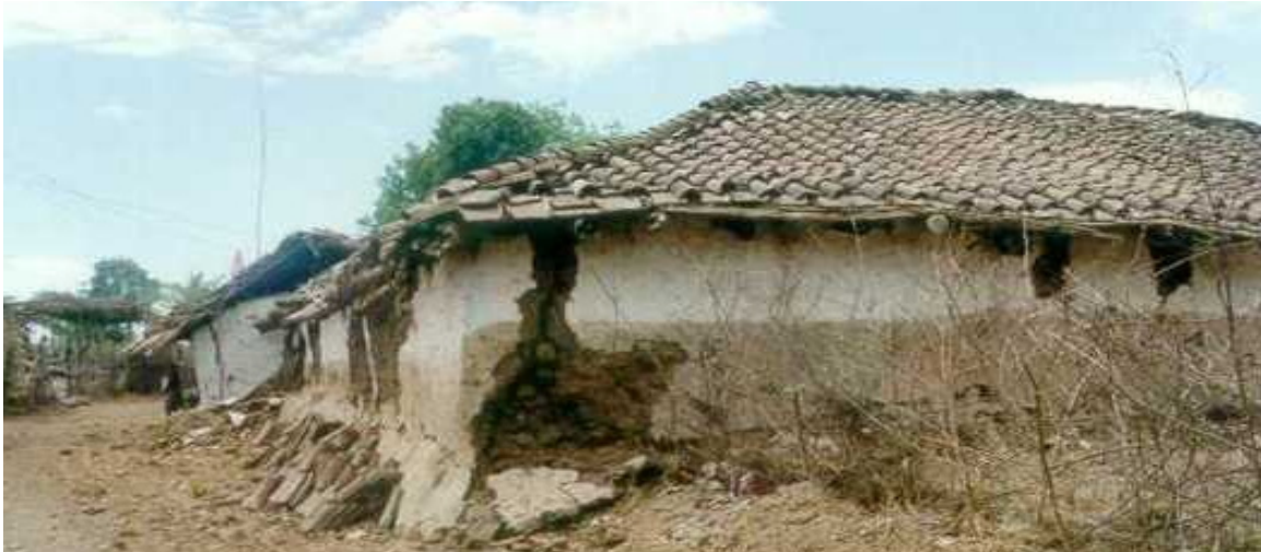
Image: Typical Earthquake Damage - Cracking and Separation of Walls in the 1997 Jabalpur Earthquake
