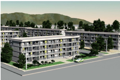
Image: Andaluçia community. First low-rise building in Chile seismically isolated by using NRB. Source: Chapeo (2011)
