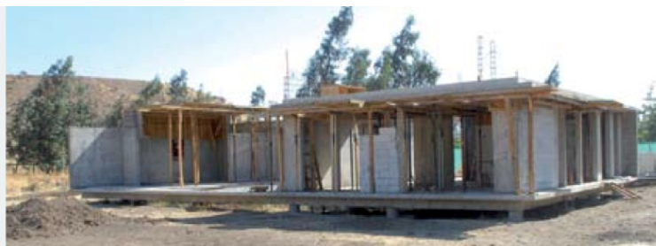
Image: Housing unit seismically isolated by using SCS Source: www.sirve.cl
