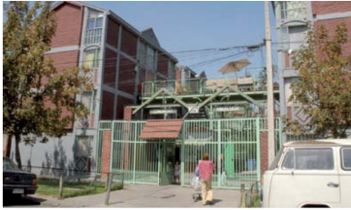
Image: Andaluçia community. First low-rise building in Chile seismically isolated by using NRB. Source: Chapeo (2011)
