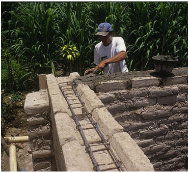
Image: Crown beam Image Source: http://www.flickr.com/photos/hawkey/3279361503/in/photo-stream/
