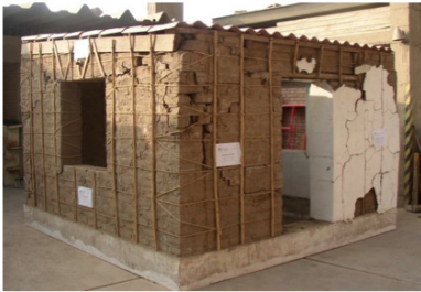
Figure 2.1.3: Internal and exterior vertical poles.
