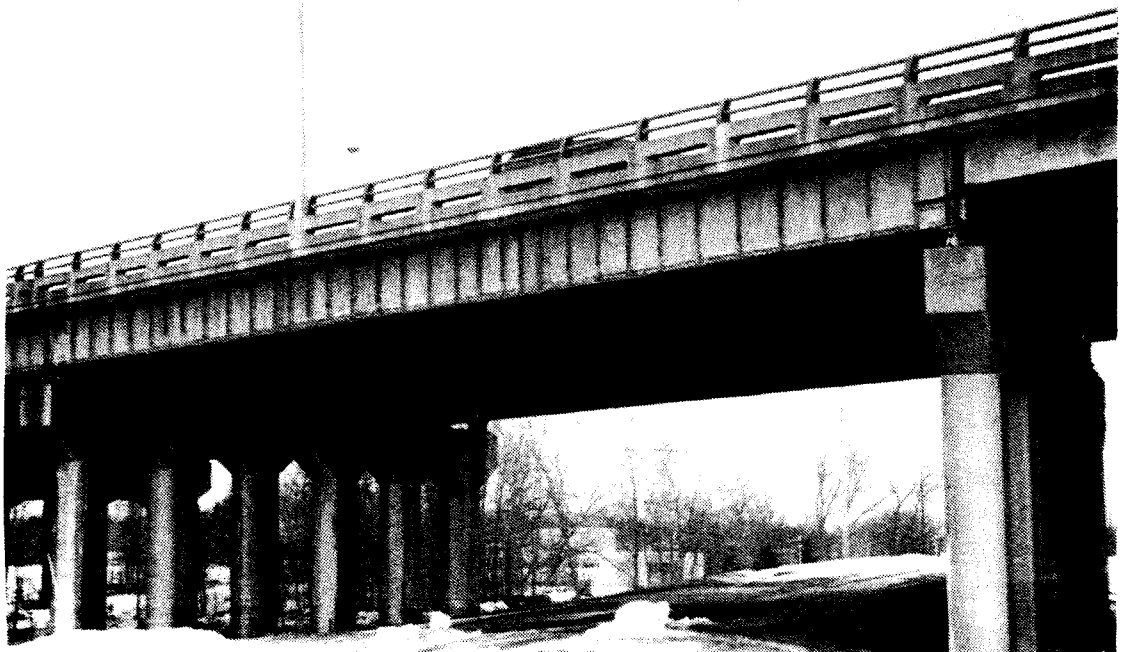
Figure 3.5 View of typical girder
