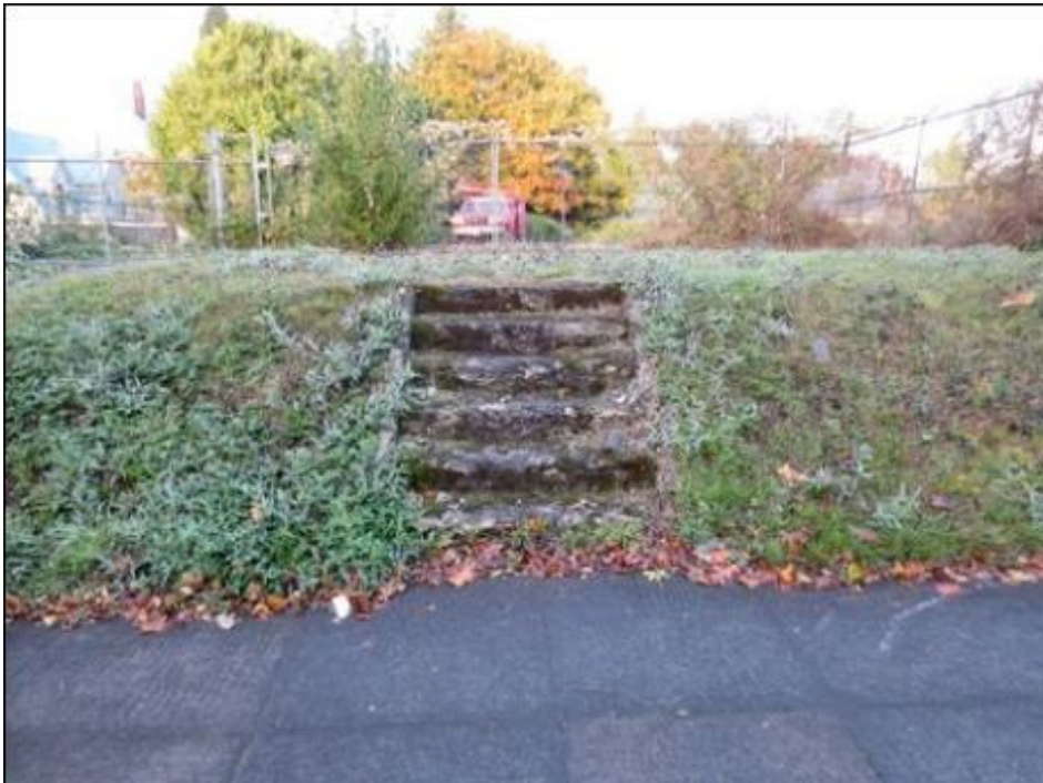
Figure 14: Steps in front of an empty lot on N. Williams Ave. north of Skidmore St. as of May 2012
