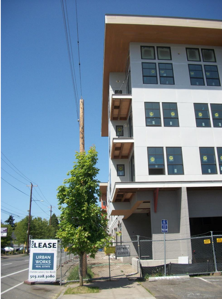
Figure 11: Condominium construction on N. Williams Ave. as of May 2012
