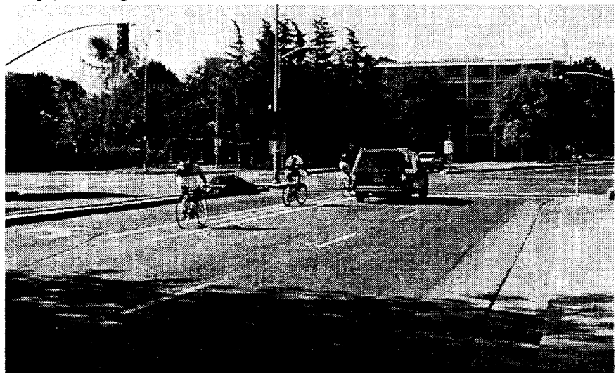
Figure 4-7. This intersection of minor arterial streets in Davis, California shows how bicycles are given equal priority with motor vehicles for making left turns. A left turn bicycle lane has been set aside (with loop detectors). Although not visible in this view, the path of the left-turning bicycles through the intersection has been painted and lined with reflector hubs.
