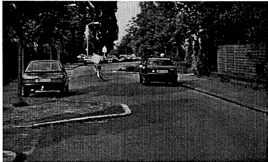
Figures 5-15 and 5-16. Traffic calming measures that force turning movements can shorten the visual length of the street for the motorist and narrow the motor vehicle's pavement.
