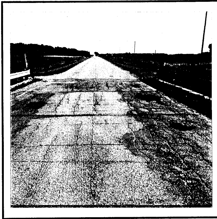
Figure 2.4 Longitudinal Pavement Crack
