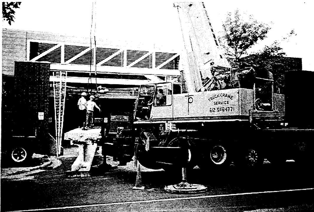
Figure 4.16 Specimen Between Crane Lifts
